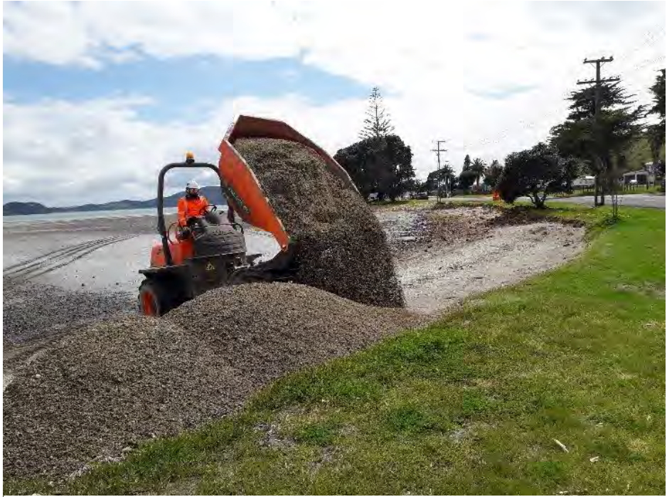
Figure 34: Cobble and sand nourishment to protect a narrow reserve along Kawakawa Bay Coast Road (Source: Auckland Council)
