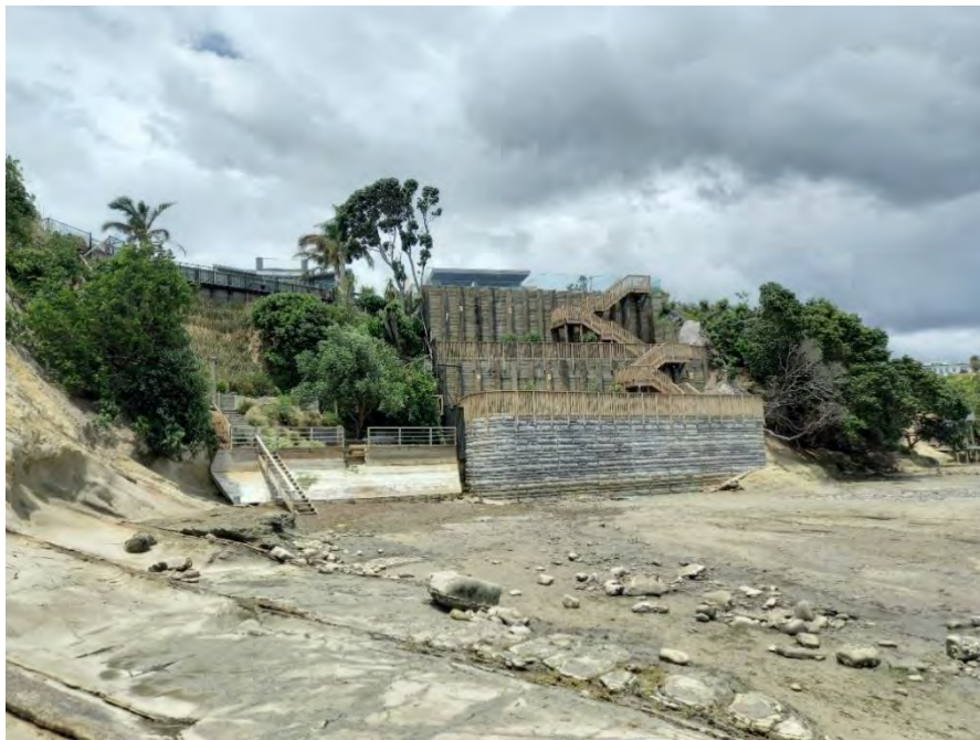
Figure 39: An example of coastal protection structures at Beachlands (Source: Auckland Council)
