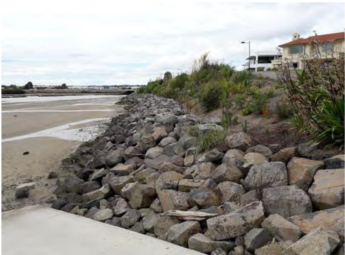
Figure 44: Karaka Harbourside - Stage one rock revetment, constructed in 2015 (Source: Auckland Council)
