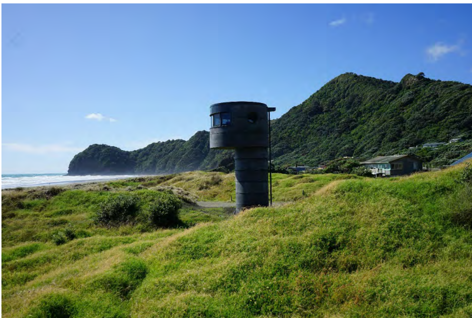
Figure 25 Te Pae Surf Tower in North Piha (Kensington, 2023).
