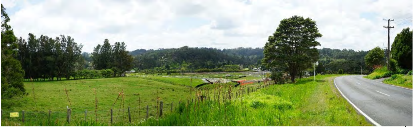
Figure 15 Looking towards the Christian Road development. The site has been cleared for construction and roads have been built (Kensington, 2023).
