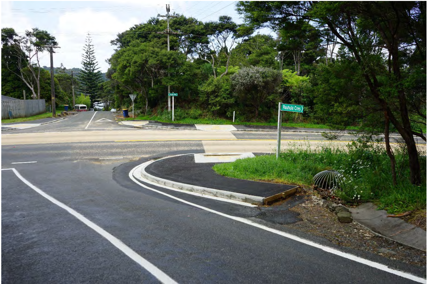
Figure 40 New roading layout at the intersection of Huia Road and Rahuia Crescent (Kensington, 2023).
