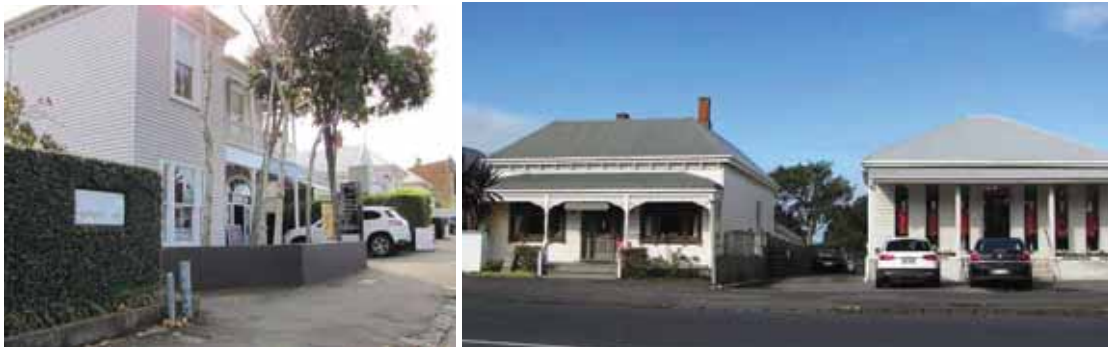
Figure 4-27. Businesses occupying residential zoned dwellings between Parnell and Newmarket
