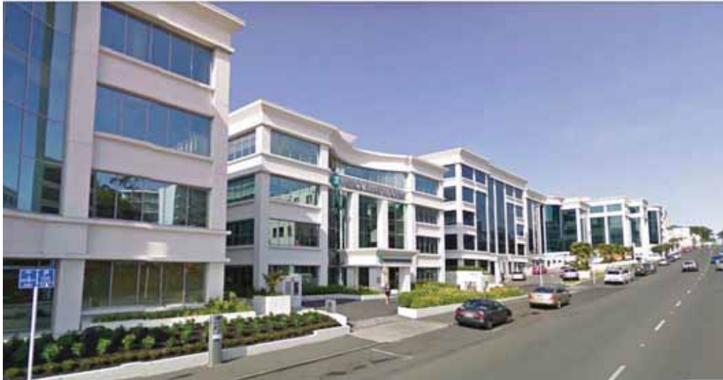
Figure 4-17. Carlton Gore Road commercial development. Source: Google Streetview
