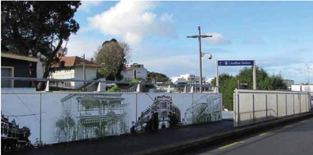
Figure 4-15. Grafton train station, Khyber Pass Road.
