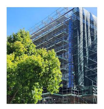
Thousands of aluminium fins are being installed onto the Wellesley entrance building's dark concrete, in a range of different colours. This upper façade design treatment is an expression of the tears of Ranginui (the sky father). The scaffolding comes down later this year.
