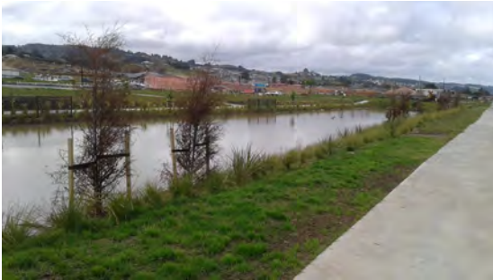
South, SHA Project Papakura Stormwater channel, SW network
