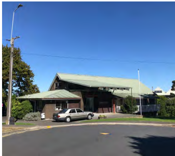
View Point 11 Facing south towards Taitamariki Hall
