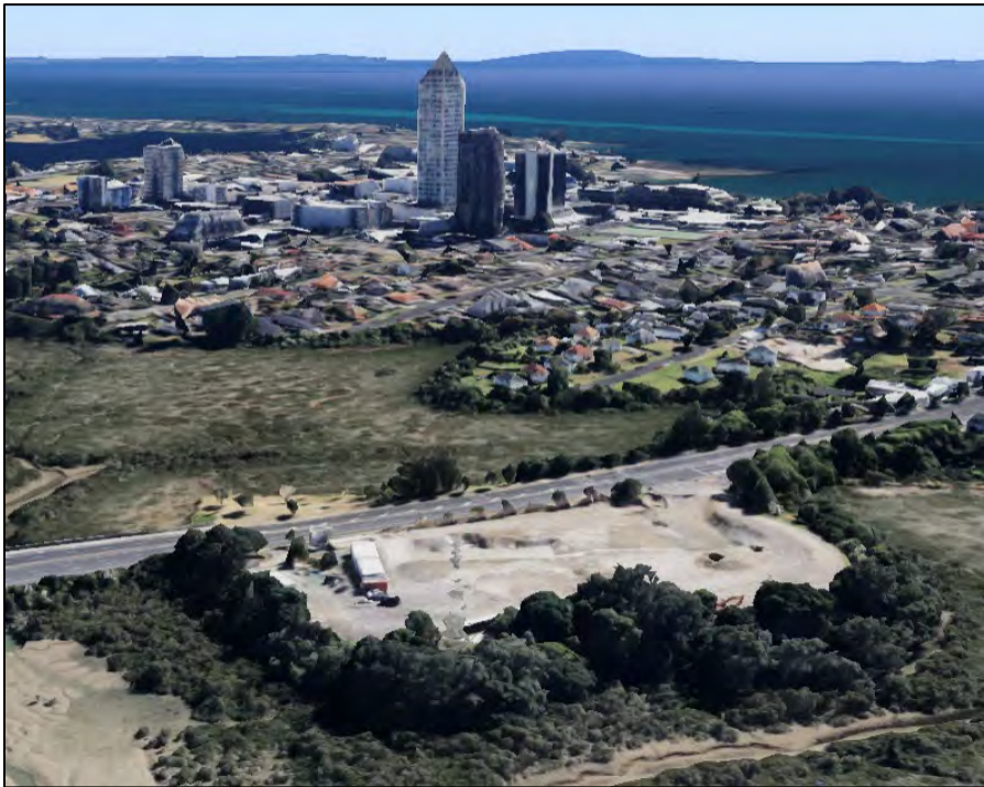
Figure 2: View of subject site facing north toward the Takapuna town centre.
