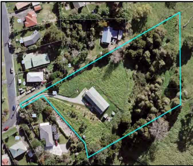
Figure 12: Aerial image of 26 Batten Street, Wellsford
