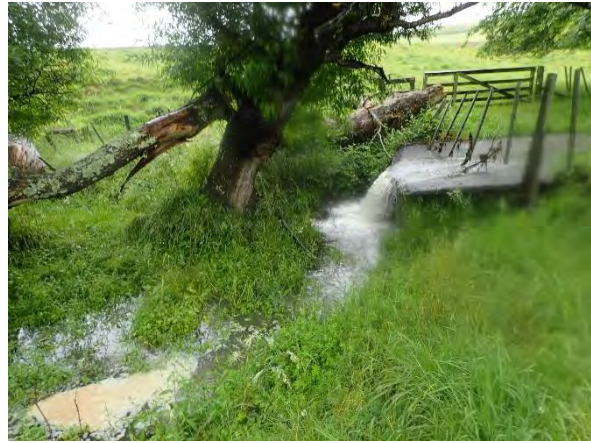
Figure 36. Weir within wetland W-B.
