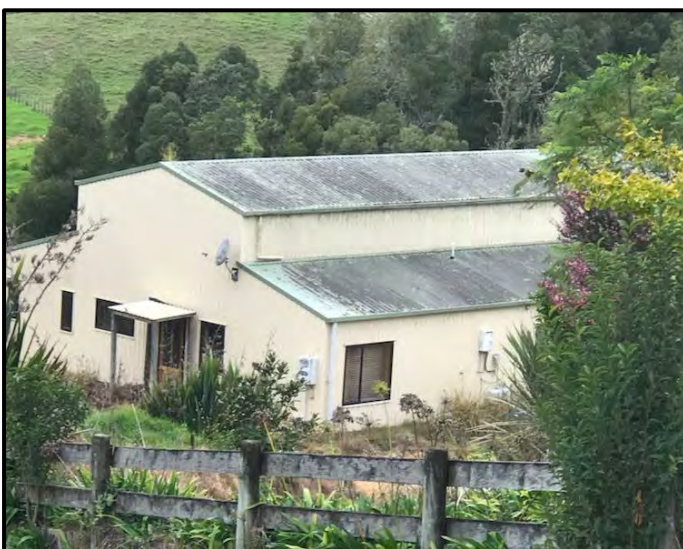
Image 5: Barn dwelling 26 Batten Street, Wellsford
