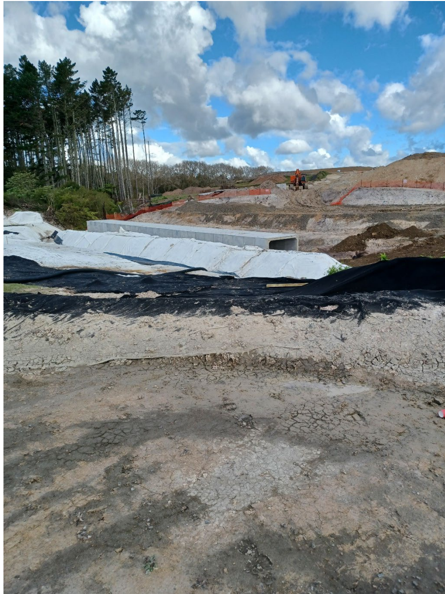
Figure 1 – Sinton Stream Culvert under construction as of 17 April 2024
