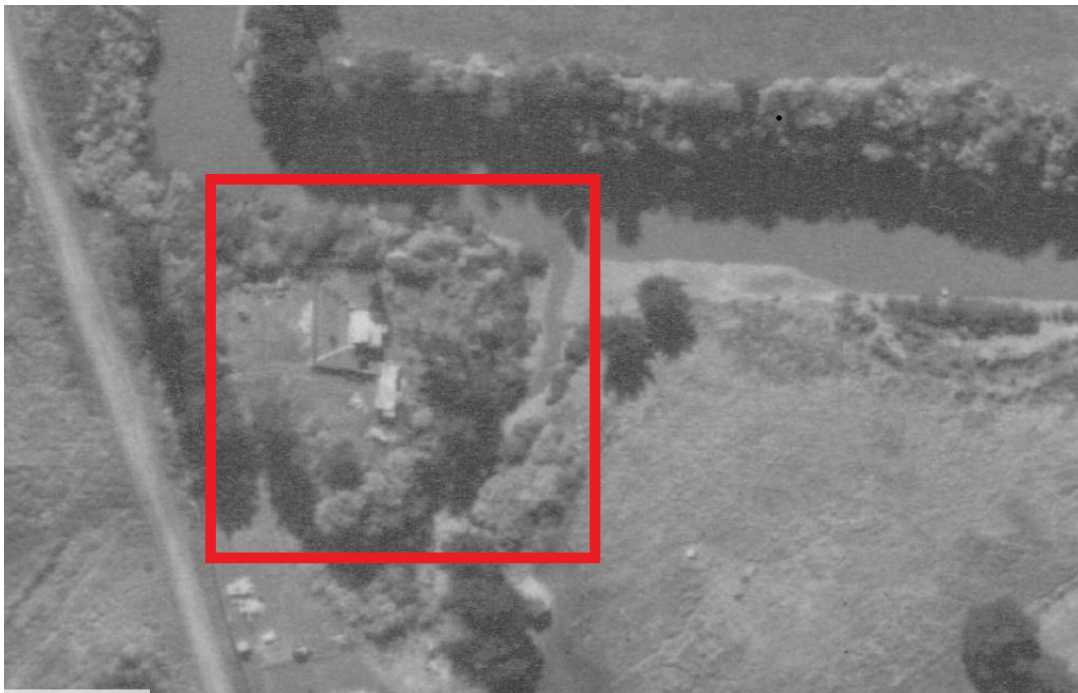
Figure 3: 502 Oruarangi Road, Mangere (1959)
