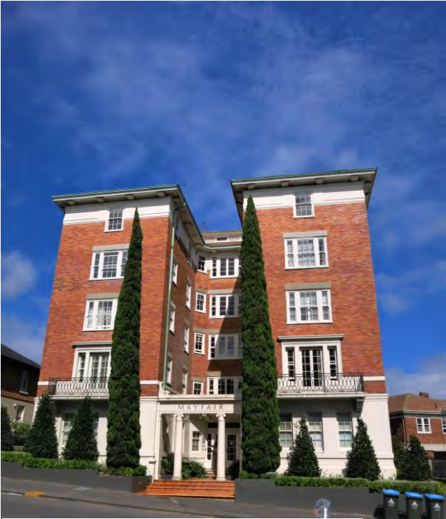
Mayfair apartment building, Parnell Road
