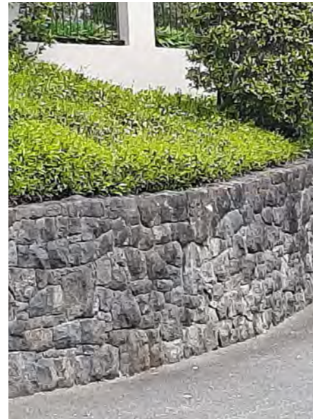
BASALT RETAINING WALL
