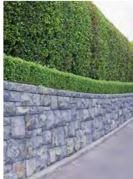
BASALT RETAINING WALL
