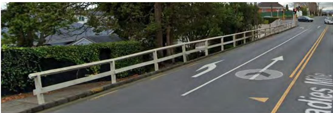
Figure 1. Existing slip lane barrier with timber fencing
