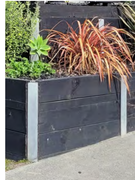
TIMBER / STEEL BEAM RETAINING WALL
