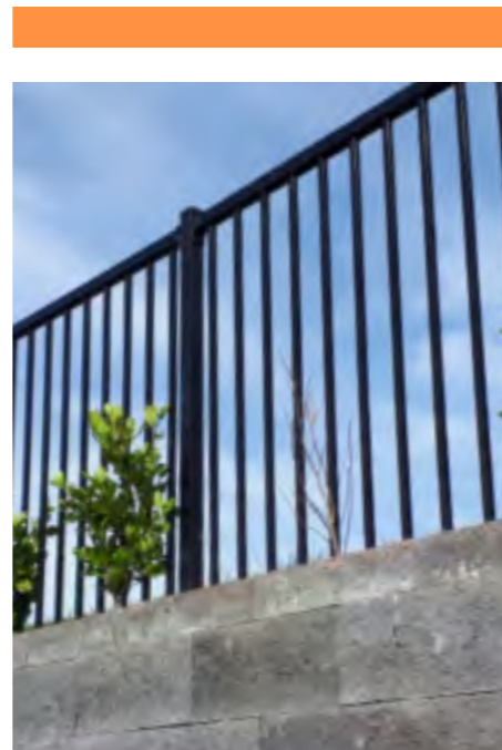
VERTICAL RAIL FENCE (F4 BALUSTRADE) - 1.2m
