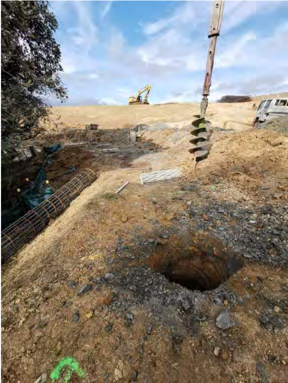
Inset 3: Construction Photos
