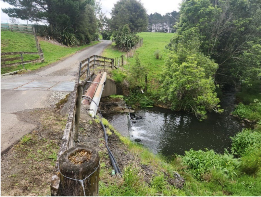
Figure 3: Downstream Extent of Bridge (18/01/2024)
