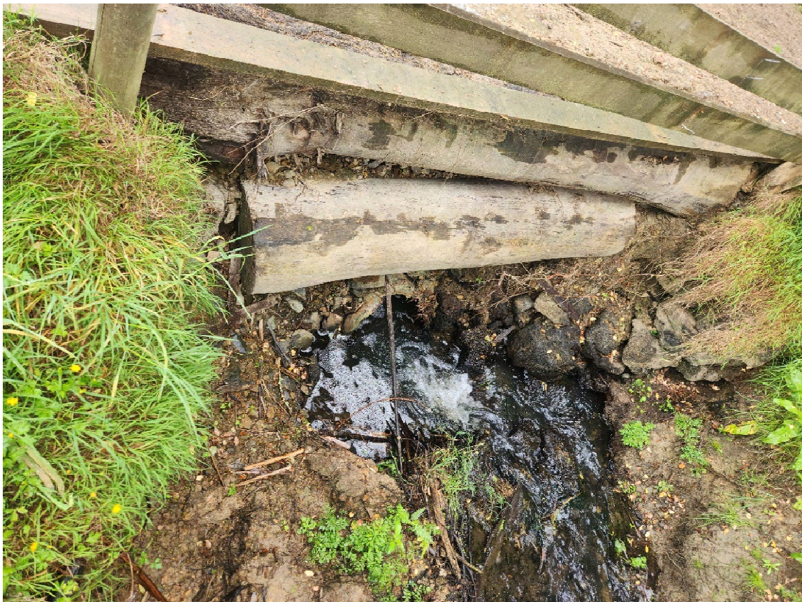
Figure F: DN 600 Culvert Inlet (06/09/2023)
