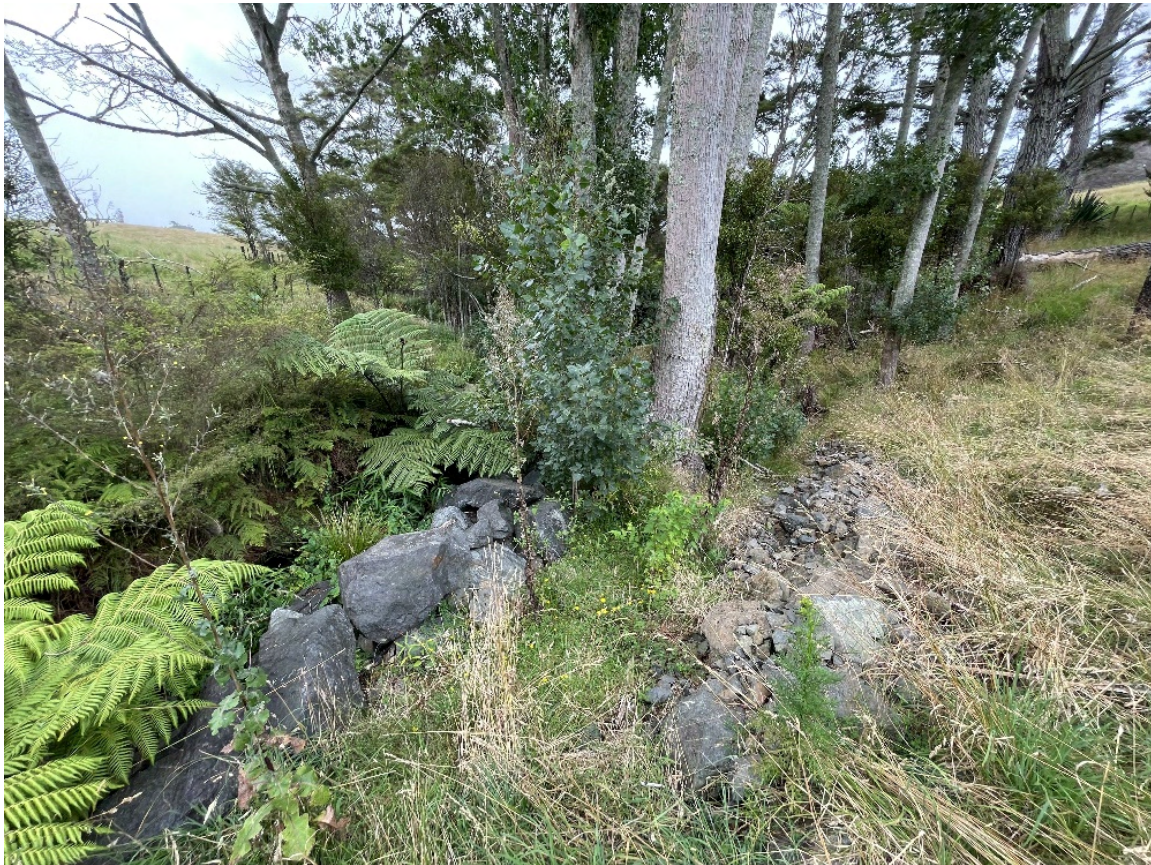
Figure D: Riprap along Stream (18/01/2024 – Facing Downstream)
