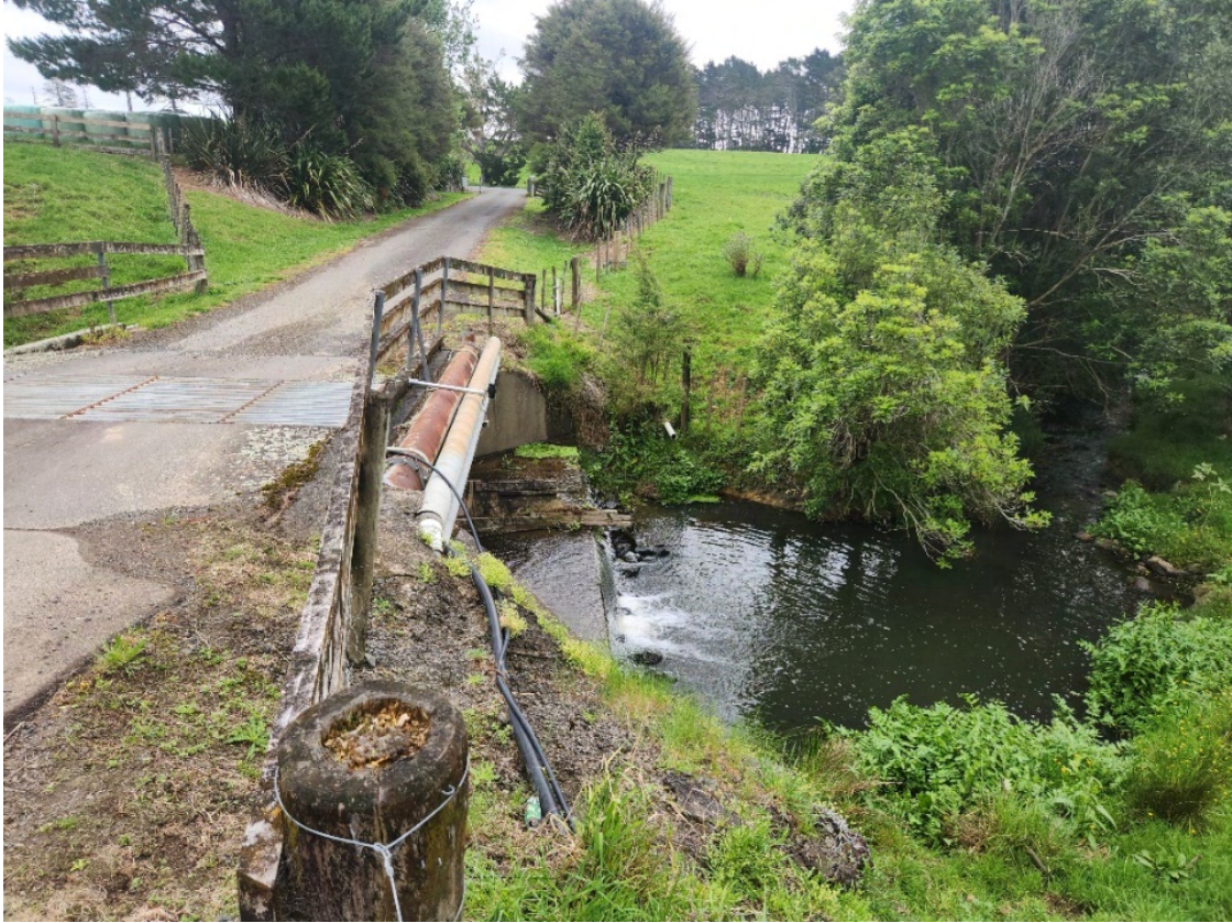
Figure I: Downstream Extent of Bridge (18/01/2024)
