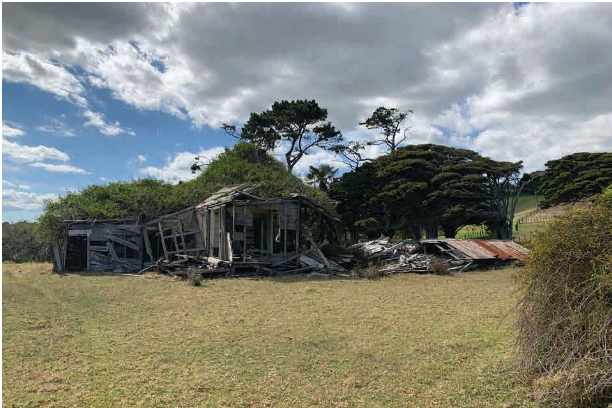
Figure 20. General view of the dilapidated cottage Q11/614, looking north.
