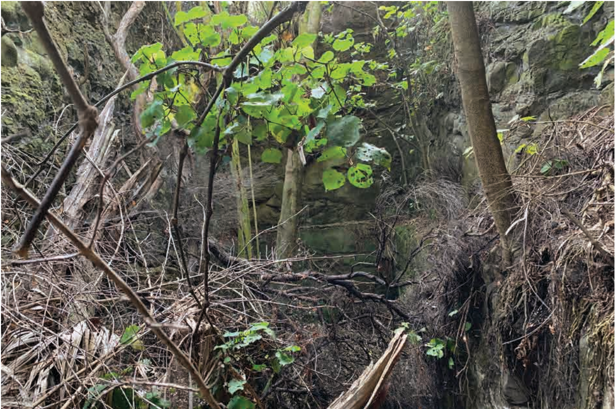
Figure 15. Overgrown vegetation in waterwheel slot, Q11/380.
