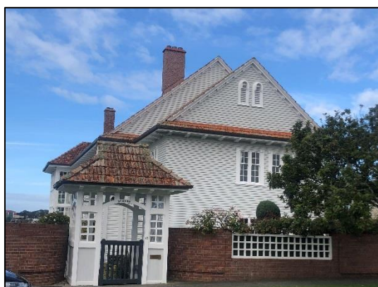
Figure 13. Existing view of street-facing façade including lych-gate. Source: DPA Architects.
