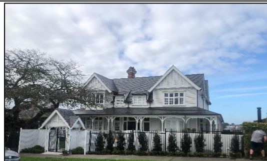
Figure 20. 9 Arney Road. Source: DPA architects.
