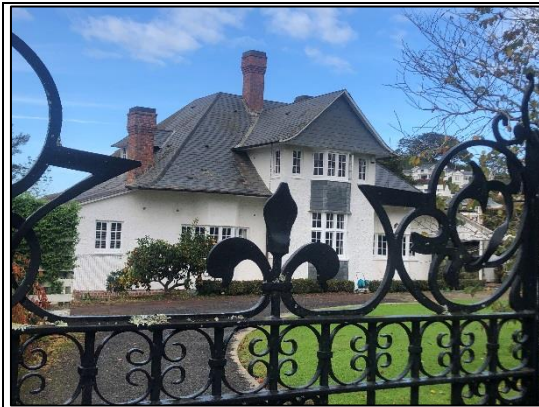
Figure 15. 11 Arney Road. Source: DPA Architects.
