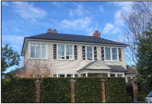
Figure 17. 51 Arney Road. Source: DPA Architects.
