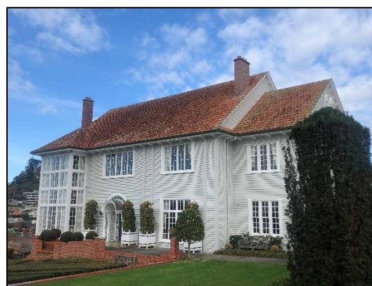
Figure 14. Existing street view of east façade. Source: DPA Architects.
