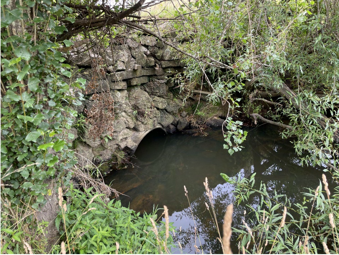
Figure K: Downstream Extent of DN 1200 Farm Culvert (18/01/2024)
