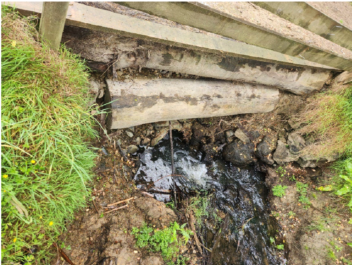
Figure F: DN 600 Culvert Inlet (06/09/2023)
