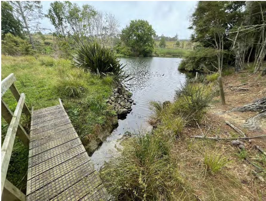
Figure 2: WWTP Discharge Pond Outlet Channel (18/01/2024)
