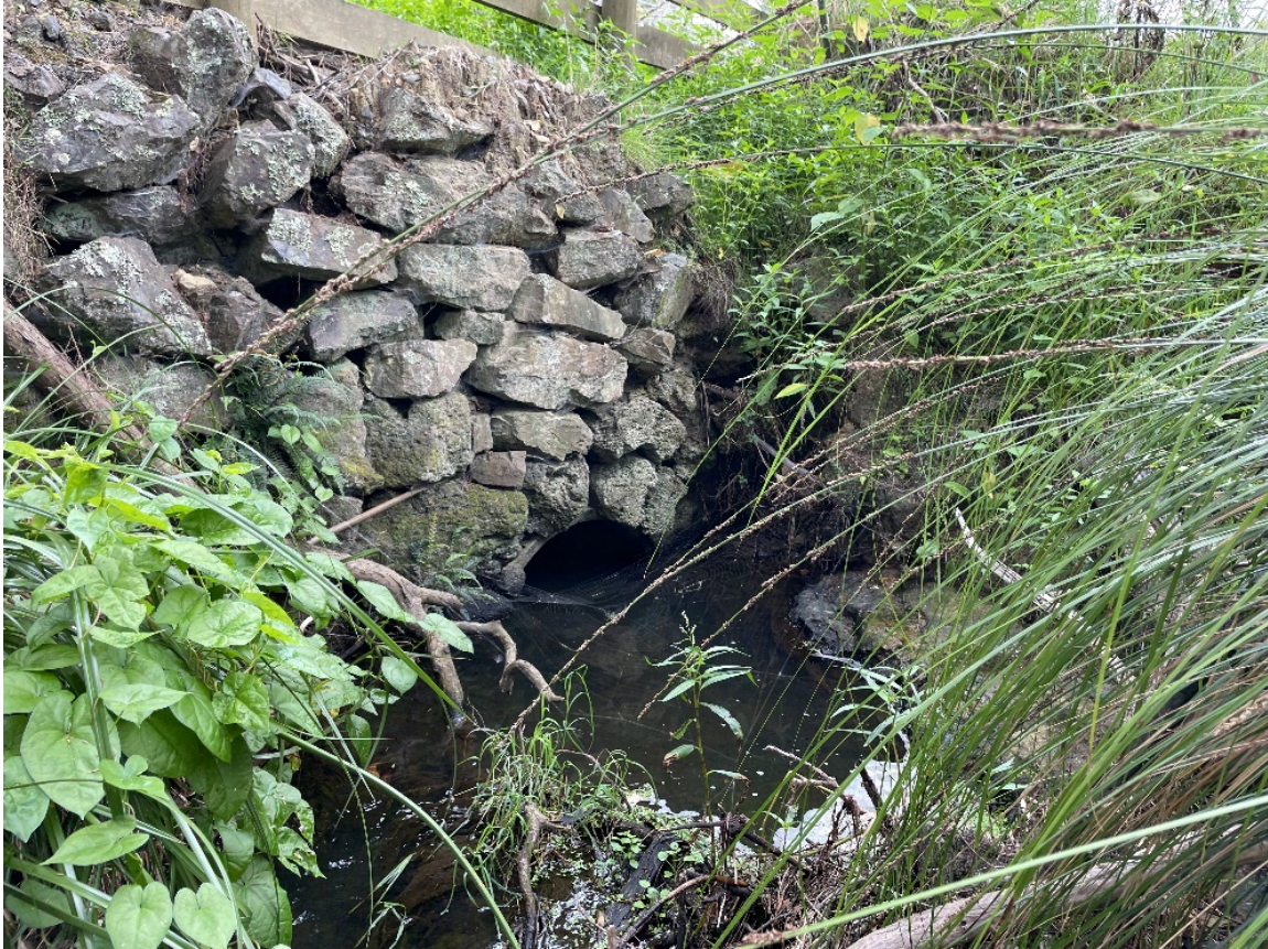
Figure G: DN 600 Culvert Outlet (18/01/2024)
