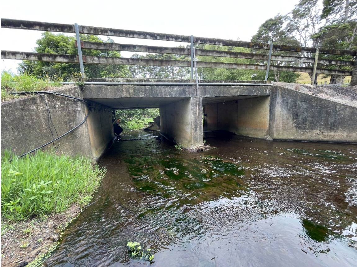
Figure H: Upstream Extent of Bridge (18/01/2024)
