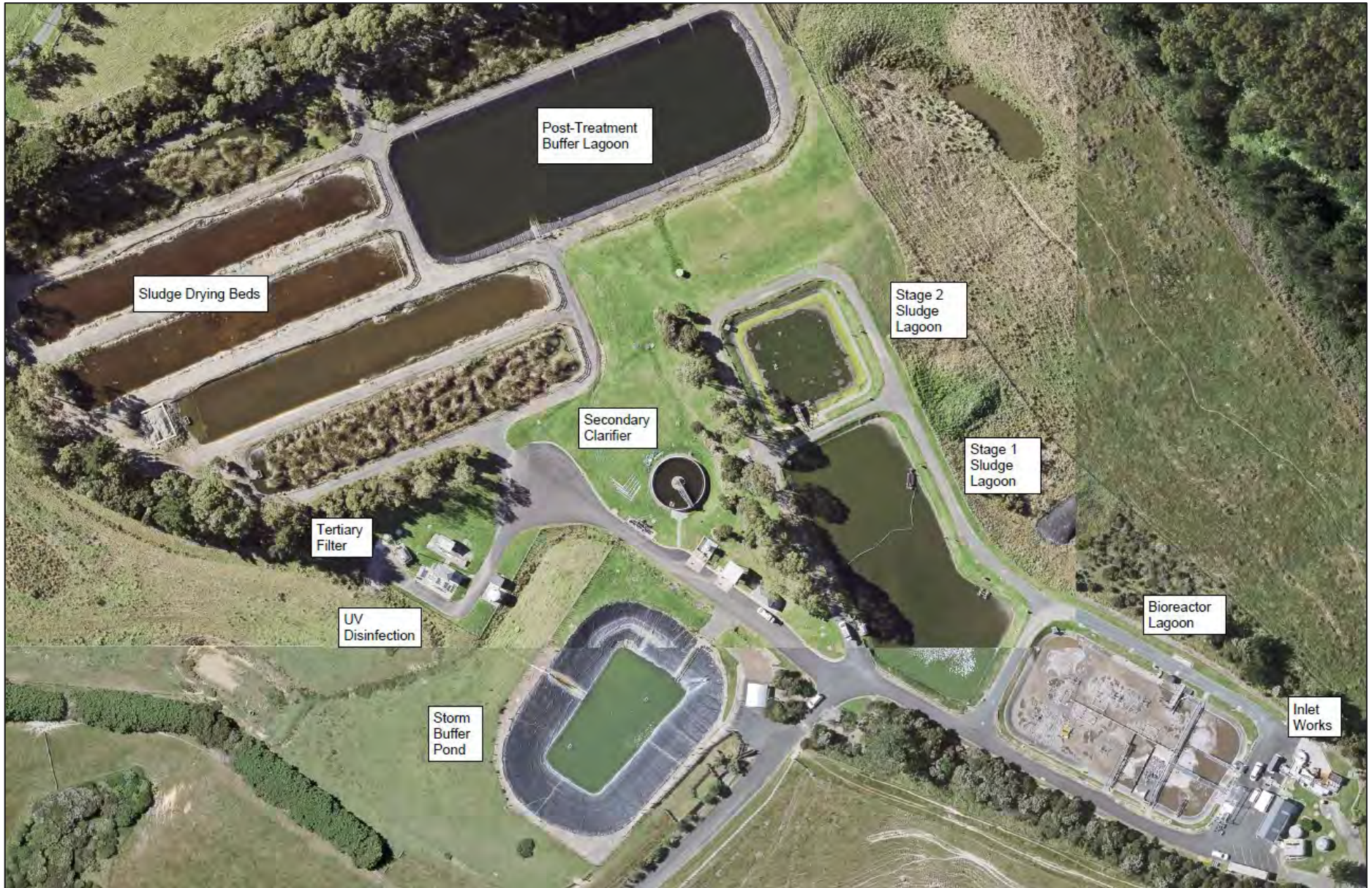
Figure 2-5: Beachlands WWTP Aerial Photograph – Current Layout
