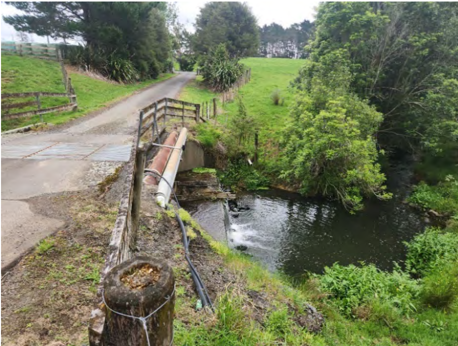
Figure 3: Downstream Extent of Bridge (18/01/2024)
