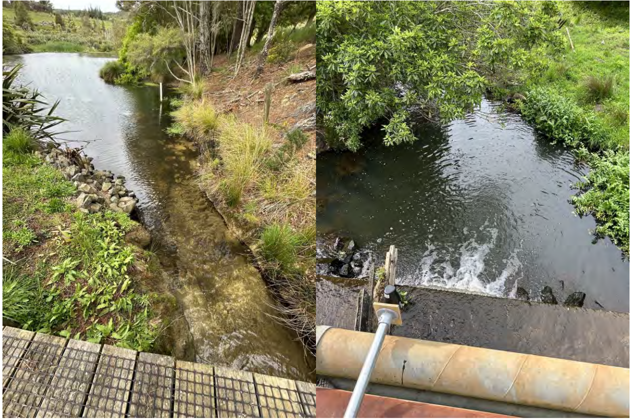
Figure 3. Farm pond (B) (left) and Bridge (15) (right) sites.
