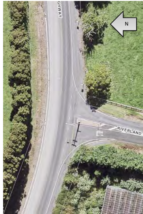
Riverland Road intersection
