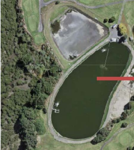
Clarks Beach WWTP Services the Clark Beach and Glenbrook Beach Communities
