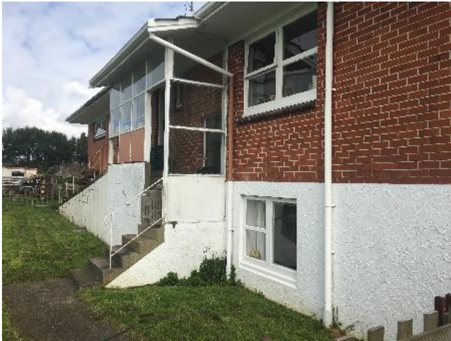
PLATE 3: EASTERN SIDE OF THE ORIGINAL DWELLING
