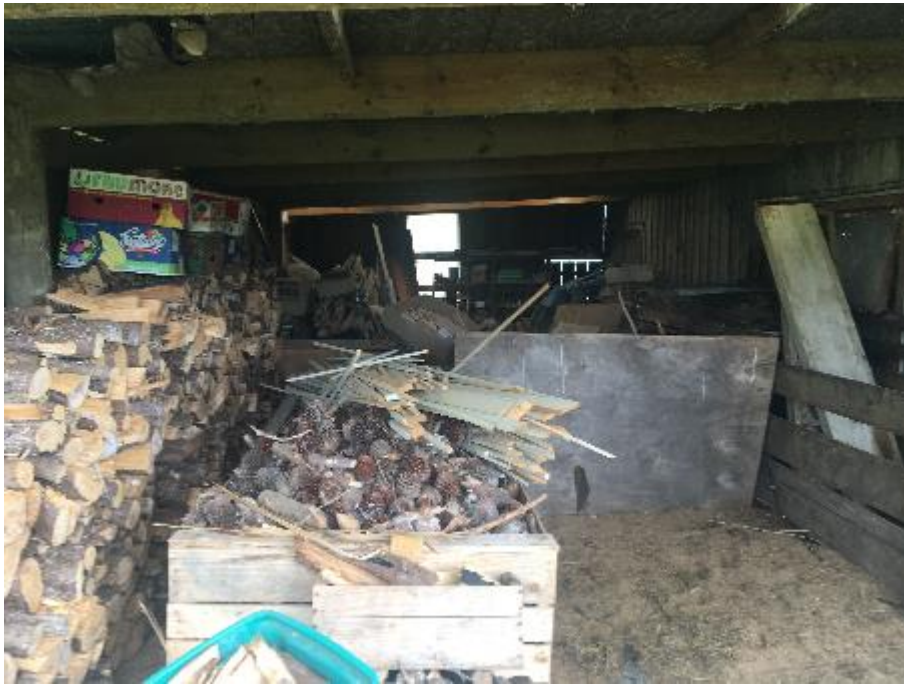
PLATE 7: INTERIOR OF BARN / TRACTOR SHED
