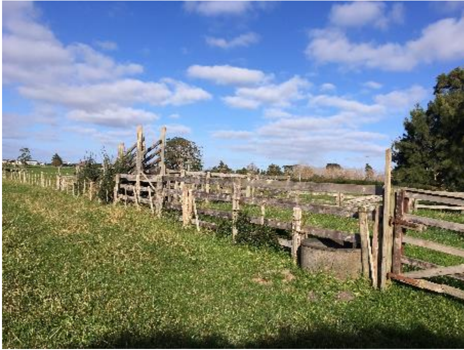
PLATE 1: LOADING BAY ADJACENT TO SITE ACCESS
