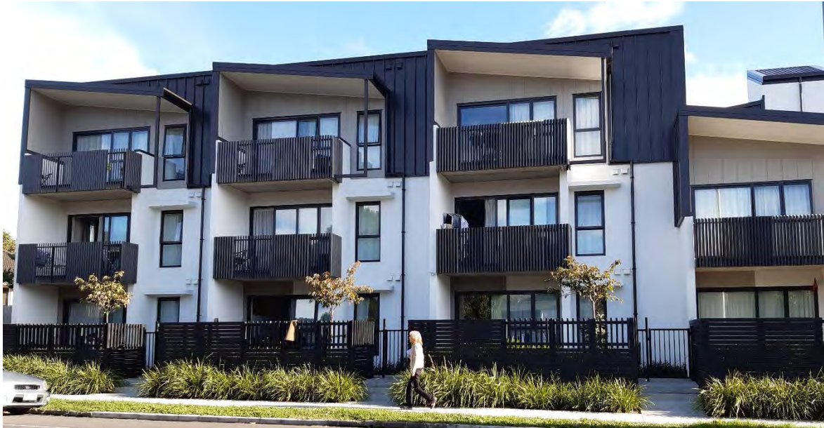
Figure 23. This development shows how privacy is achieved for the ground level apartments when there is a height separation and landscaping between the primary outdoor living area and the public footpath.
