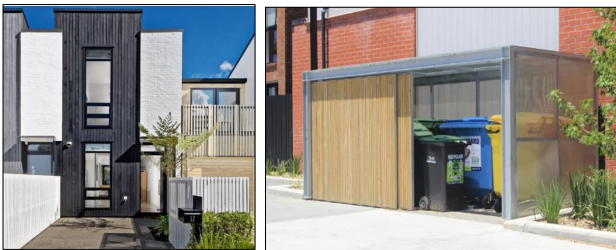
Figure 35: The left image shows a white fenced enclosed area to the right of the property which visibly screens the waste bins from the street while maintaining convenient access for residents. This dwelling is in Hobsonville where developments comply with design requirements set by the Hobsonville Land Company (now Kainga Ora). This requires rubbish bins be sited so as not to compromise outdoor living courts, be visually obtrusive and to be out of the view from the street. The right image shows communal waste bins stored in a well designed, ventilated, easily accessible communal waste area with good access for residents and on-site waste collection.
