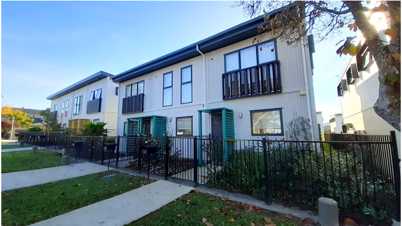
Figure 10: A wide street frontage enables rows of terraces to face the street with individual entrances and landscaping. Short building lengths and spaces between buildings enable daylight to more rooms within dwellings.
