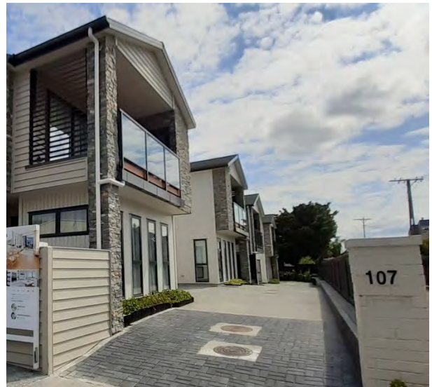
Figure 17. This development has dwellings with the principal living outlook spaces and outdoor living area in the form of a balcony at the first level overlooking their driveway towards adjoining sites – poor quality outlook and reduced privacy for residents and neighbours.
