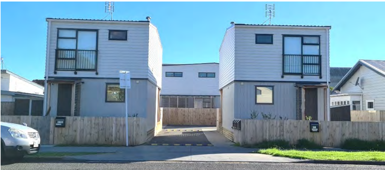
Figure 5: The limited width of this site influenced the number of street facing dwellings and the site arrangement of buildings around vehicle access and parking areas. The central driveway is the primary access to rear carparking and a row of terraces at the rear of the site.
