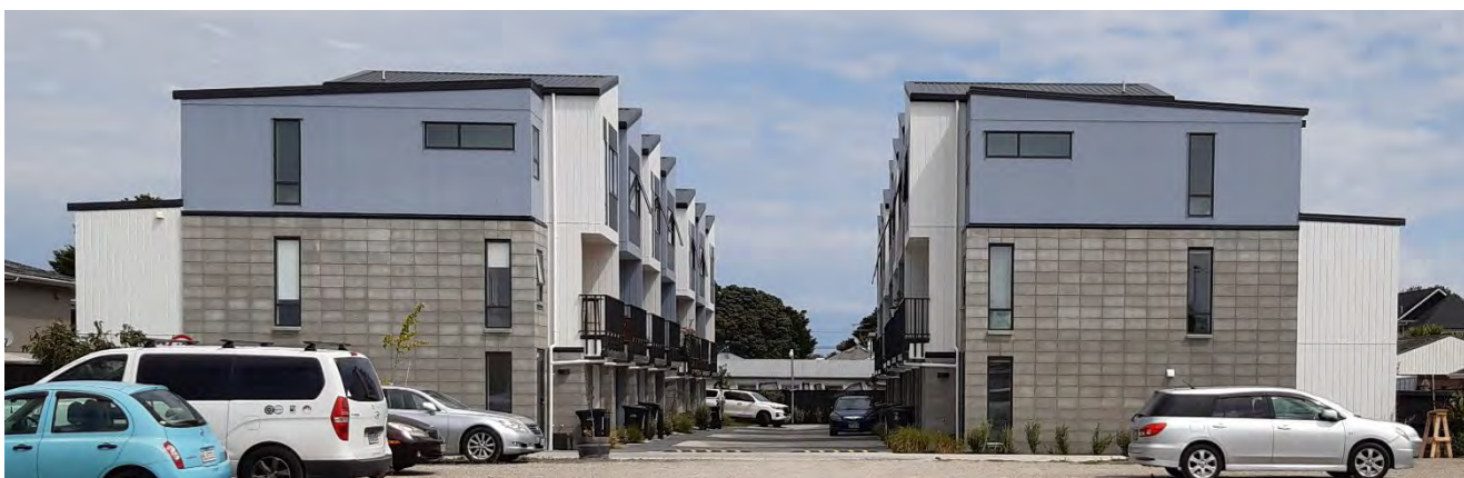
Figure 18. This three storey terrace development shows the outdoor living spaces (in the form of a balcony on the first level) and principal outdoor living space taking advantage of the driveway space to meet the AUP standards. The AUP requirement for sunlight to outdoor living spaces plus the requirement for a 6m outlook space from the living area has caused the 6+m wide driveway to be located in the central core of the development. The outlook spaces and outdoor living spaces (balcony) of each terrace block face each other across the driveway which can affect privacy.
