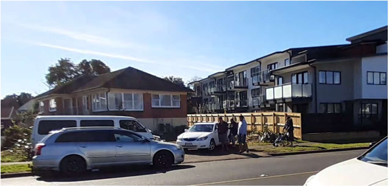
Figure 22: Three storey apartment development with complying outdoor living areas in the form of balconies and ground level courtyards facing the boundary may affect privacy on the adjoining site.
