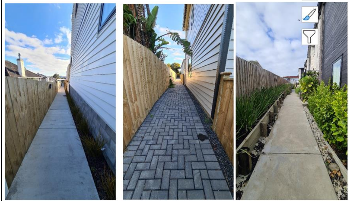
Figure 25: 0.2m to 1m separation distances between pedestrian accessways and dwellings (Source: pg. 37 of the TMDO report).
