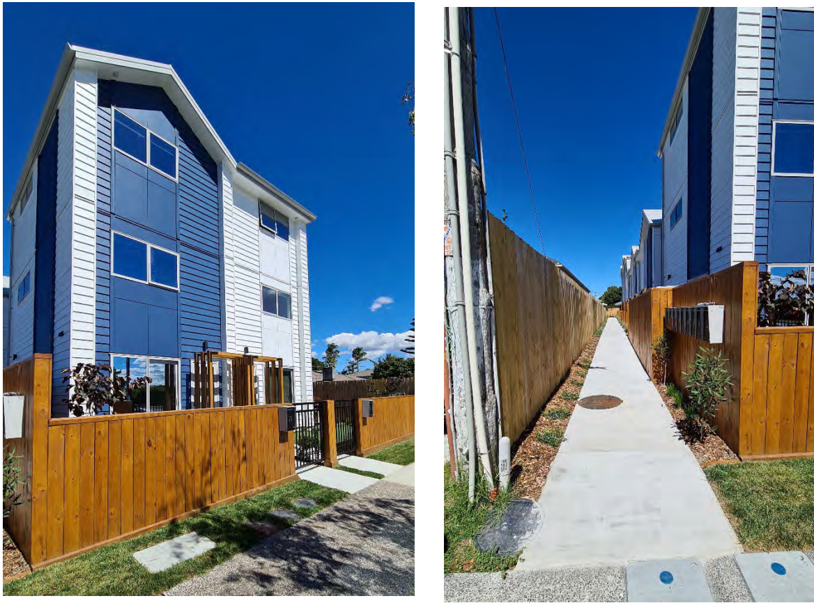
Figure 9: This 11 dwelling terrace housing development on a 809m 2 site in the THAB zone has a site width of 15m and 54m depth. There is no on-site parking, so a footpath provides access to dwellings and the majority of terraces face the adjoining site. There are three buildings of different lengths - 6.5m, 21.4m, 17m with two spaces of 1m and 1.4m between the three buildings.
