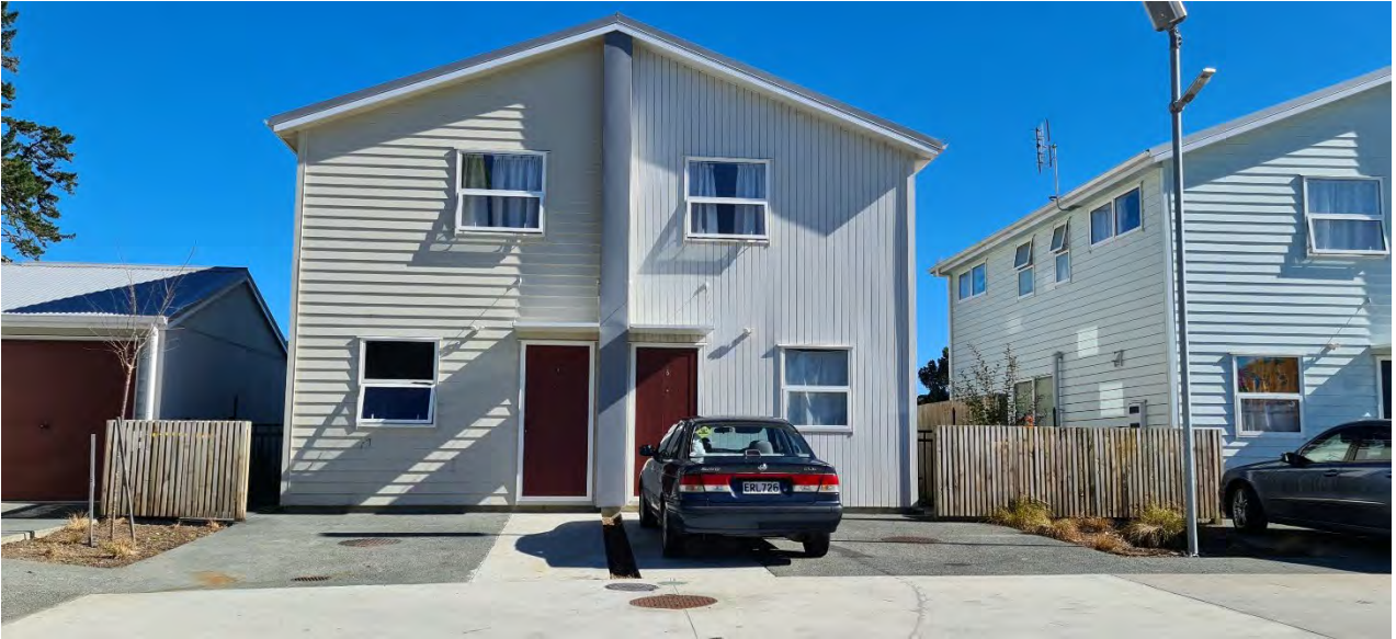
Figure 28: Observations from site visits showed poor quality landscaping and ongoing maintenance was an issue for many developments.
