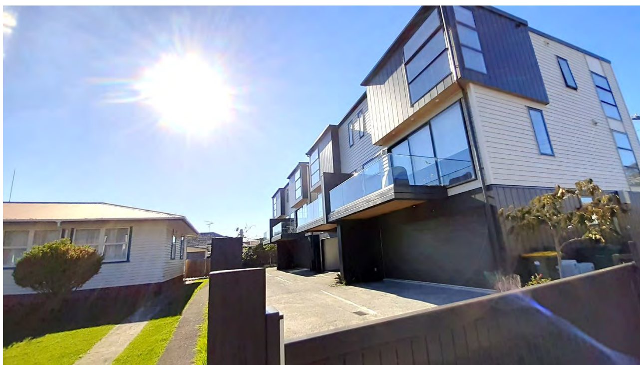
Figure 11: This development has four dwellings with the principal living area and outdoor living space in the form of a balcony at the first level, overlooking their driveway and facing the adjoining site.
