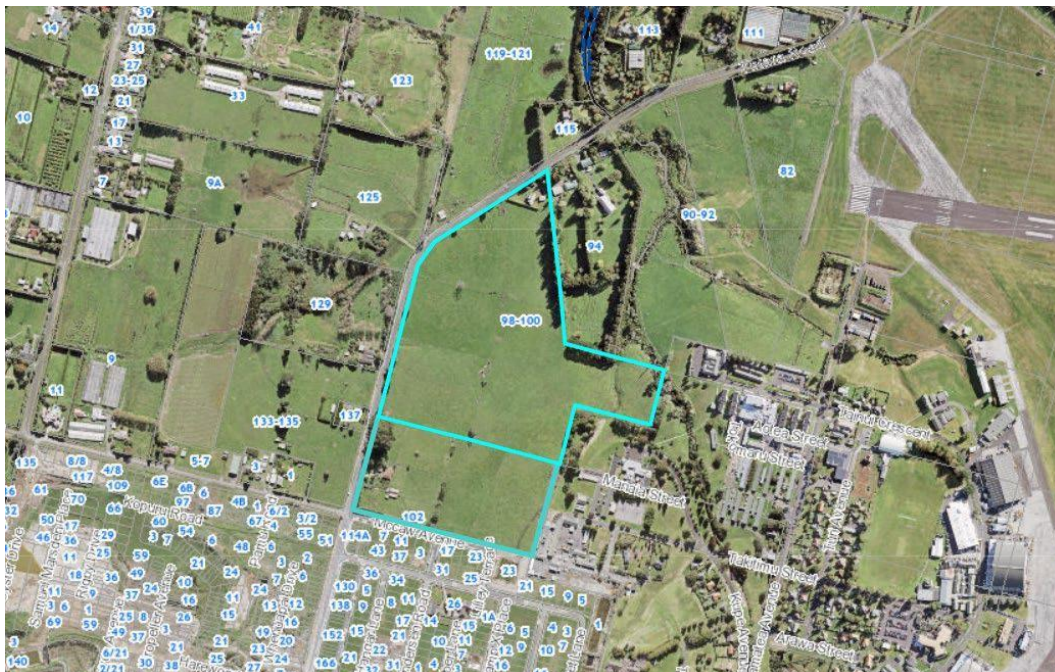
Figure 1: Aerial photo of the site at 98-100, 102 Totara Road, Whenuapai, Auckland (encircled in blue) - (Source; Auckland Council GIS)
