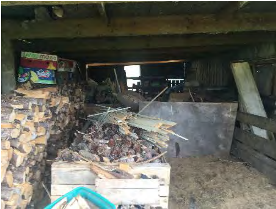
PLATE 7: INTERIOR OF BARN / TRACTOR SHED
