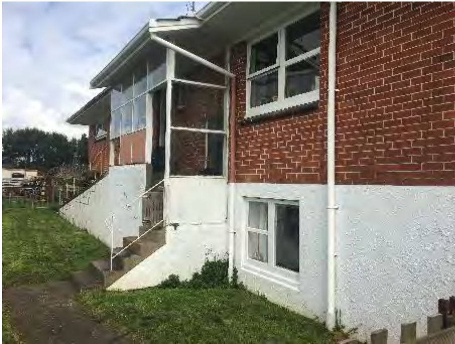
PLATE 3: EASTERN SIDE OF THE ORIGINAL DWELLING
