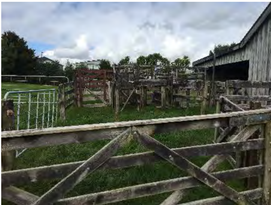
PLATE 6: PENS SURROUNDING THE BARN / TRACTOR SHED
