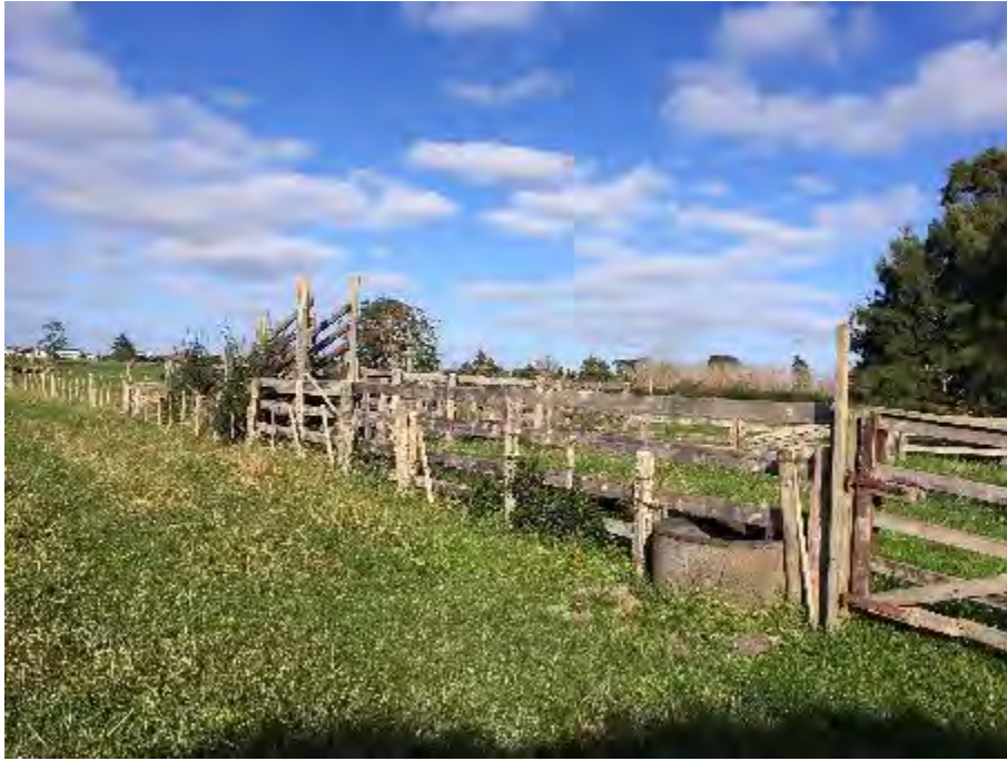
PLATE 1: LOADING BAY ADJACENT TO SITE ACCESS
