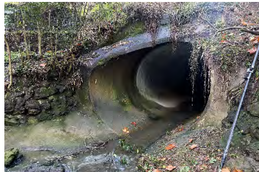
Figure: 6-2: Existing Totara Road DN2300mm culvert (view from downstream end)
