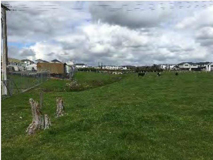
PLATE 7: STORMWATER FLOWPATH IN SOUTHEAST CORNER OF SITE, ADJACENT TO AIRBASE
