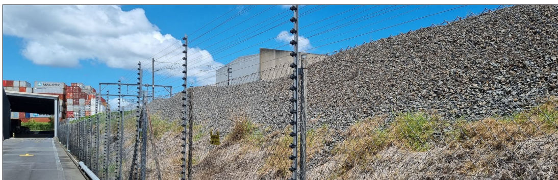
Figure 3: View looking south along the western boundary / interface with the adjoining rail corridor.
