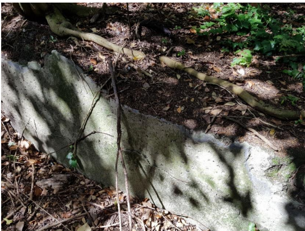
Figure 22. Close-up of one wall showing pecked surface (usually a preparation for plastering)
