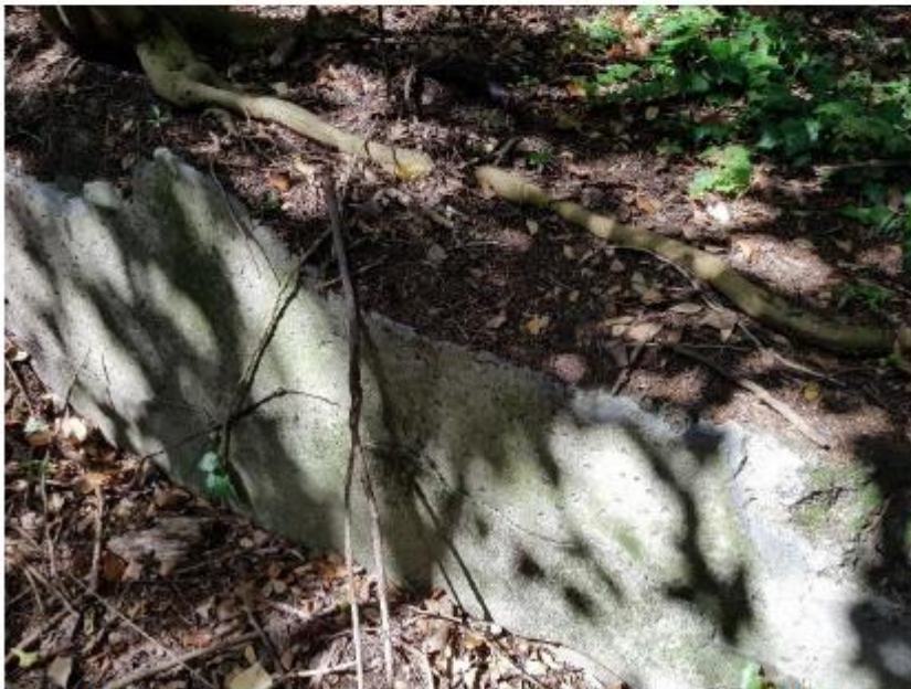
Figure 2. Close-up of one wall showing pecked surface (usually a preparation for plastering)
