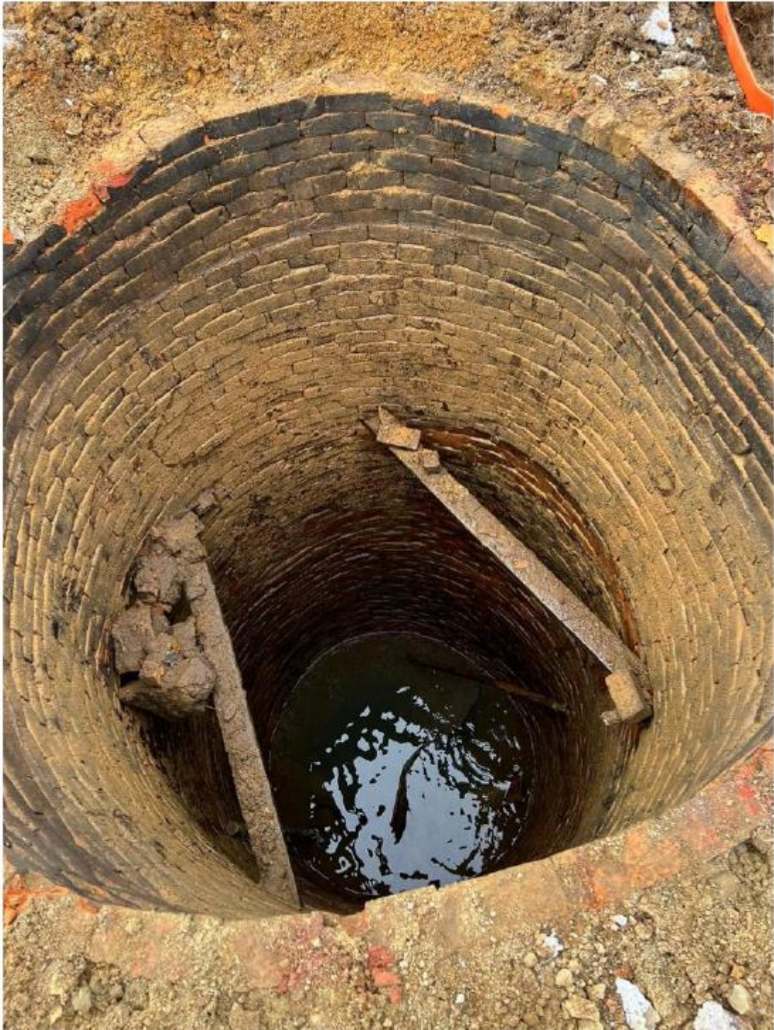
The well after draining
