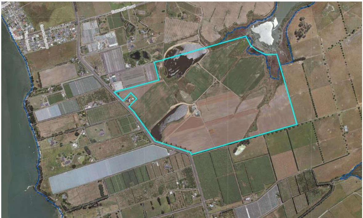
Figure 1: WWTP site and surrounds
