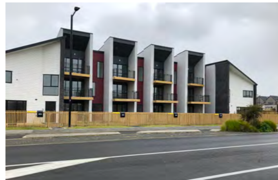
Medium density housing delivered as part of a Special Housing Area for 650+ sites, the town centre and neighbourhood park along with transport upgrades.
