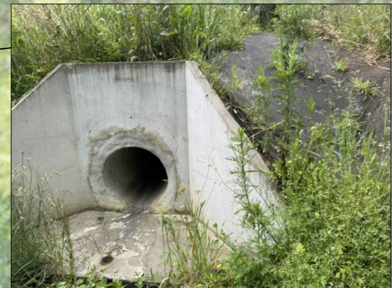
STORMWATER OUTLET - PHOTO 2
