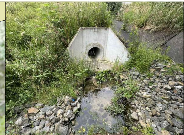
STORMWATER OUTLET - PHOTO 1
