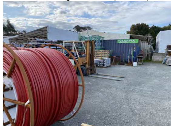
#14 Cable Storage – Traffix (Yard 13)
