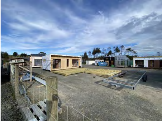
#6 Portable building construction (Yard 5)
