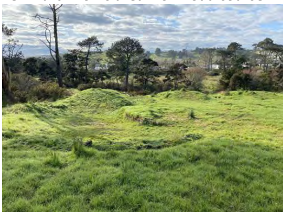
#8 – Earthworks area – off-road course
