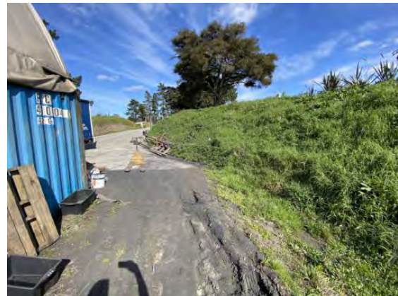
#27 – sand on W side of shed
