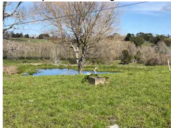
#7 – Treatment pond with earth bund
