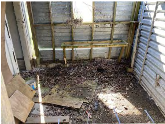
#1 – Inside lean-to shed
