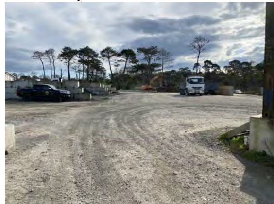
#5 Aggregate soil and concrete yard
