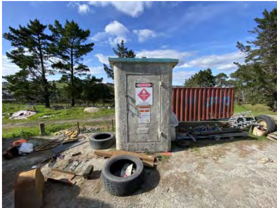
#22 – Dangerous goods store
