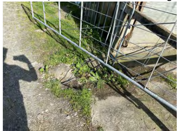
#19 – Drain on NE side of shed/stable
