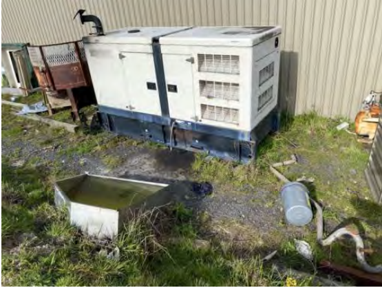
#6 Compressor on west side of shed
