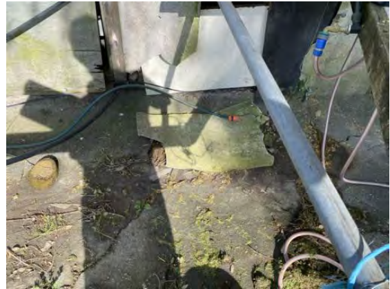
#19 – Shed/stable (broken fibrolite)
