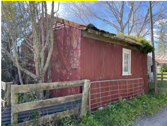
#1 – Shed with wooden floor
