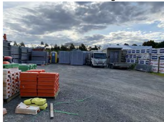
#11 Scaffold & Timber Storage
