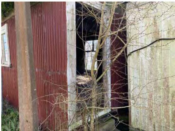
#1 – Shed with wooden floor
