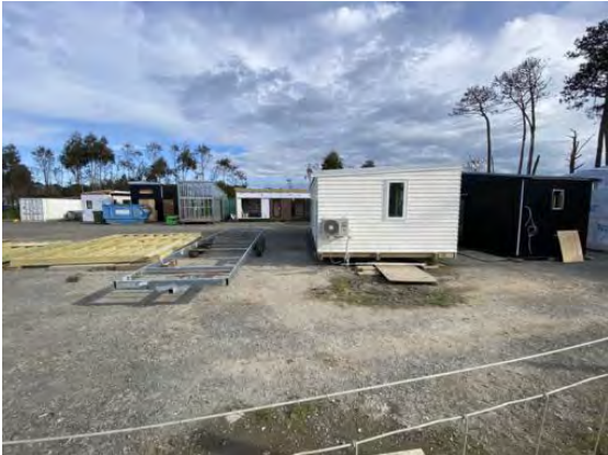
#6 Portable building construction (Yard 5)
