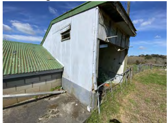
#5 – Vat room fibrolite cladding
