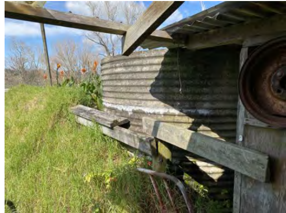
#5 – Water tank on SE corner of shed
