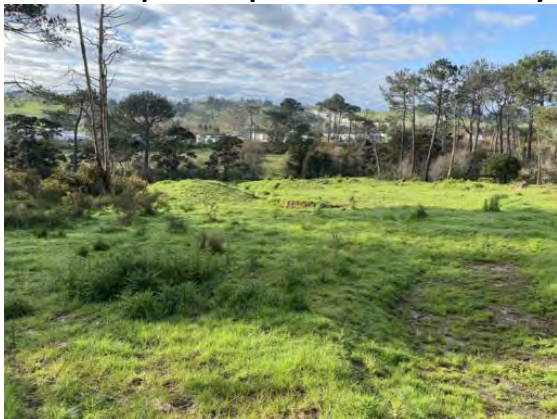
#8 – Earthworks area – off-road course
