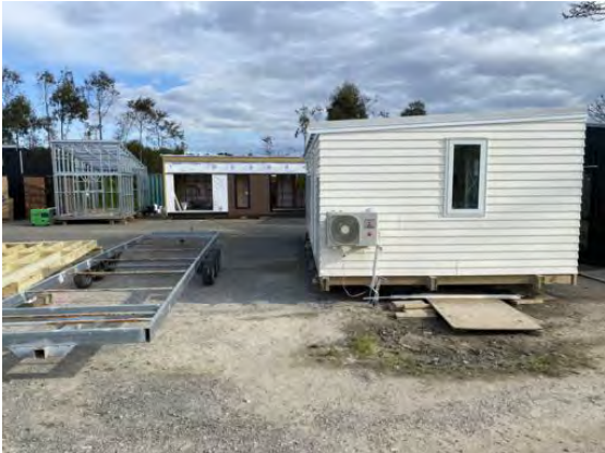
#6 Portable building construction (Yard 5)
