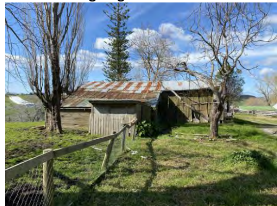
#2 GI farm sheds with earth floors
