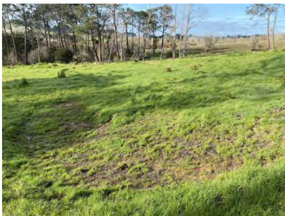
#8 – Earthworks area – off-road course
