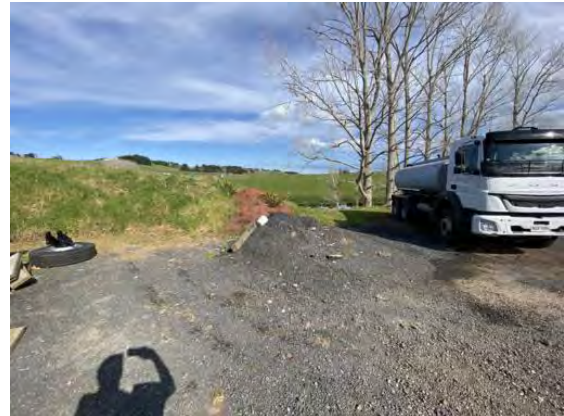
#3 Asphalt stockpile & bund edge
