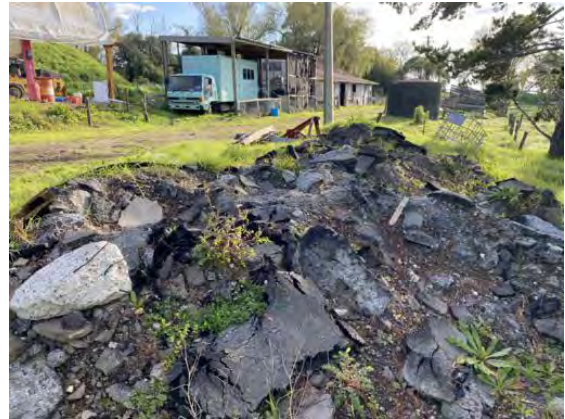
#3 Asphalt, concrete & gravel stockpile/fill area
