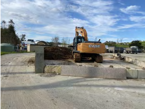
#5 Bunded soil store (Yard 5B)
