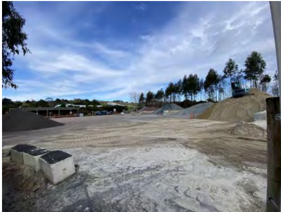
#16 Sand & aggregate depot
