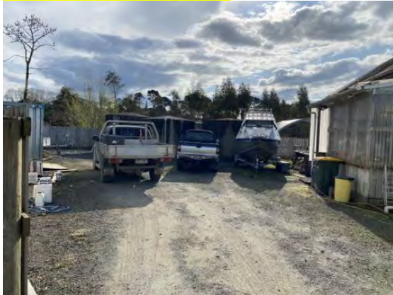
#1 Concrete water tanks SW of dwelling
