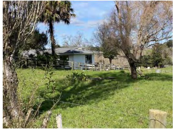
#15 Dwelling in northwest of property
