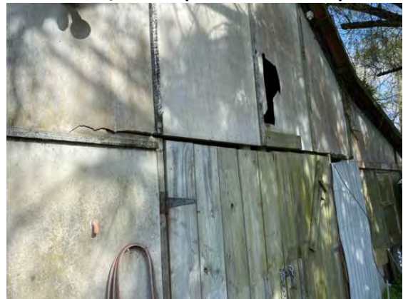
#19 – Shed/stable with fibrolite cladding
