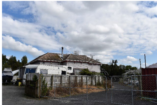
Fig. 60 Looking west showing a portion of the eastern elevation and the undated addition central to the elevation.
