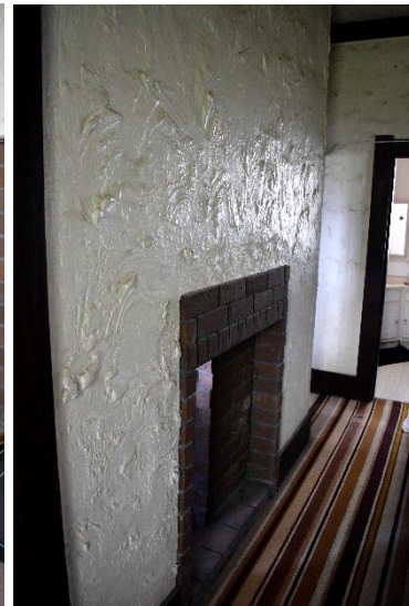
Fig. 52 An opening in the lounge allow heat from the fireplace to travel to the hallway and bedrooms. Note stucco finish on the walls, possibly added during the 1984 alterations.
