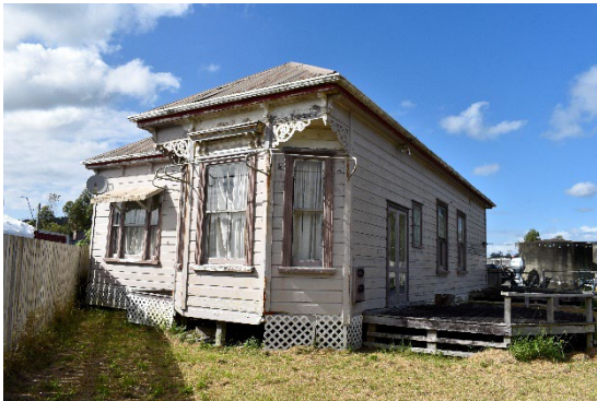
Fig. 57 Looking south towards the principal elevation of the villa.
