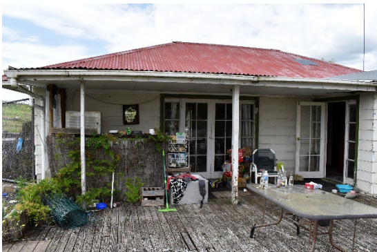
Fig. 41 Looking southeast toward the 1984 addition.
