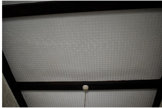
Fig. 49 A close up of the patterned lining within the hallway.
