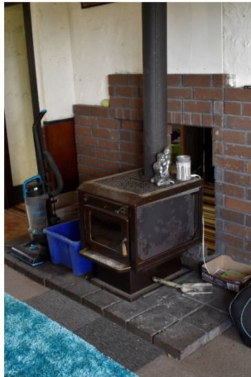
Fig. 51 The fireplace within the original lounge was installed during the 1984 alterations. Historical imagery confirms the original dwelling did not have a fireplace.
