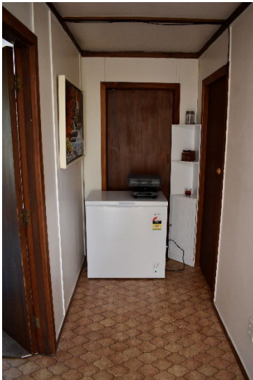
Fig. 55 Hallway of the 1984 addition.
