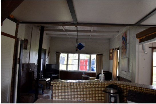
Fig. 46 Looking towards the lounge within the original portion of the dwelling,
