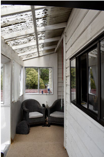
Fig. 43 Exterior rear wall of the original dwelling, closed in following the 1984 addition.
