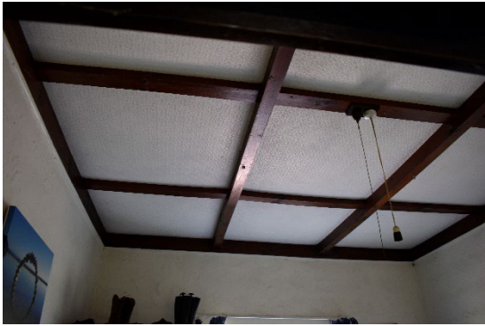
Fig. 48 Dark stained timber battens with patterned linings decorate the rooms within the original portion of the dwelling.
