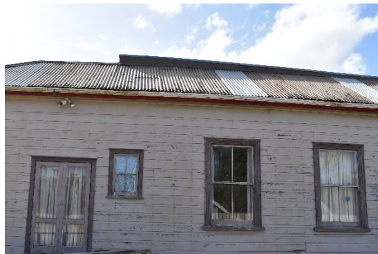
Fig. 67 The modified roof with through section sheet metal.
