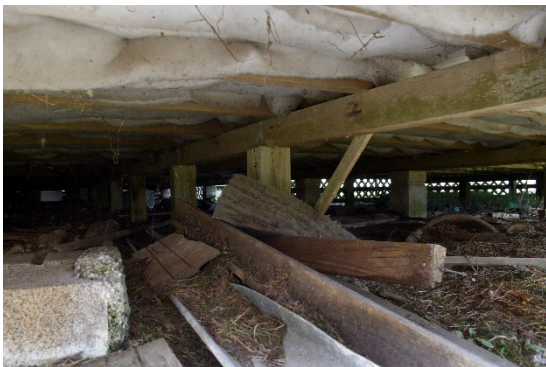
Fig. 66 Modern timber and concrete piles.
