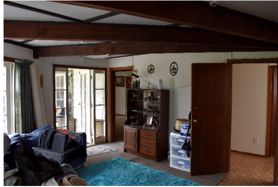
Fig. 54 Looking towards the 1984 addition from the original portion.
