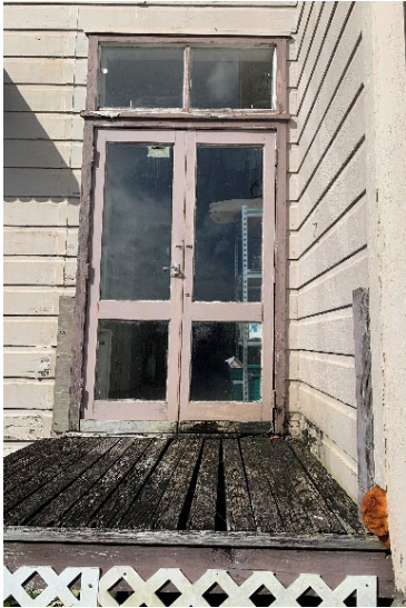
Fig. 68 Modified front door on the principal elevation.
