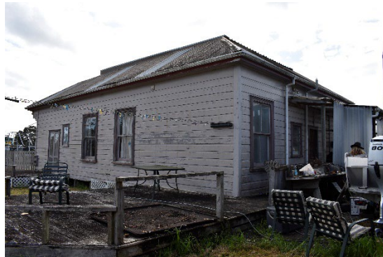
Fig. 58 Looking east towards the side elevation showing large traditional sash windows.
