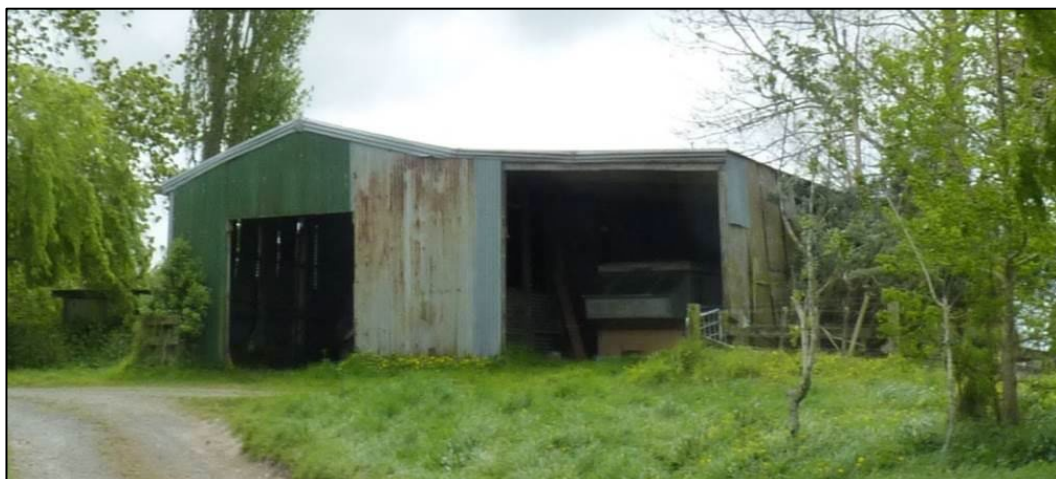
Figure 33. View of garage / shed at 1636 Dairy Flat Highway
