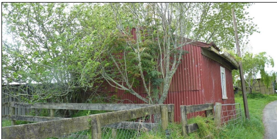
Figure 34. View of small outbuilding at 1636 Dairy Flat Highway
