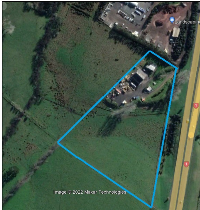
Figure 65. Property 4 image indicating extent of the modified area, and area of low-lying pasture forming the southern half of the property
