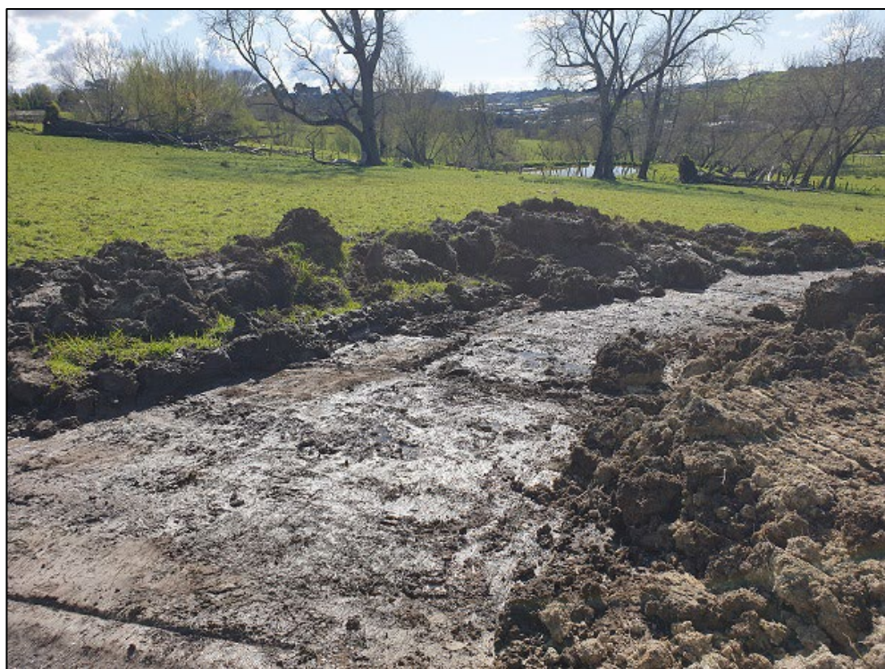
Figure 48. Cut access track with dark brown waterlogged topsoil spoil visible
