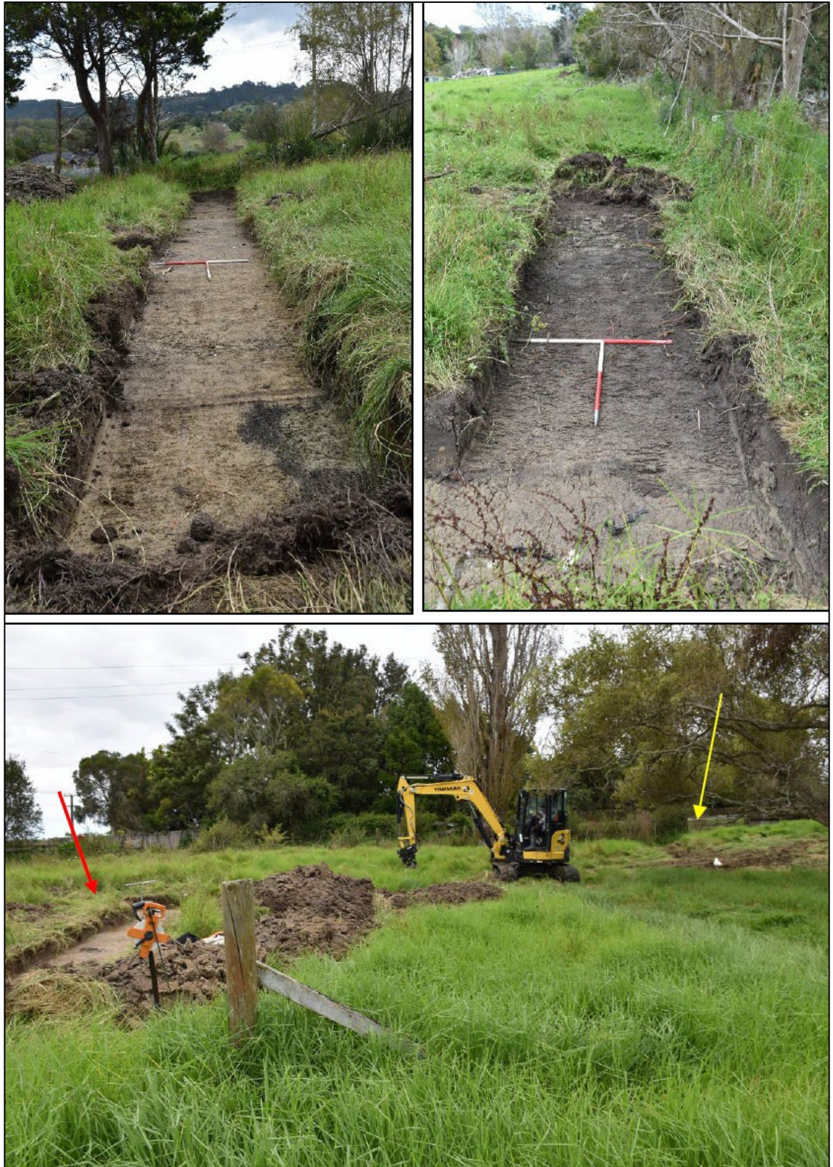
Figure 82 Trench 6 – longest trench on top left, facing north; short trench by road frontage on top right; and Trench 6 with postholes on the left (red arrow) and backfilled Trench 5 on the right (yellow arrow), facing northeast (1m scale bars)
