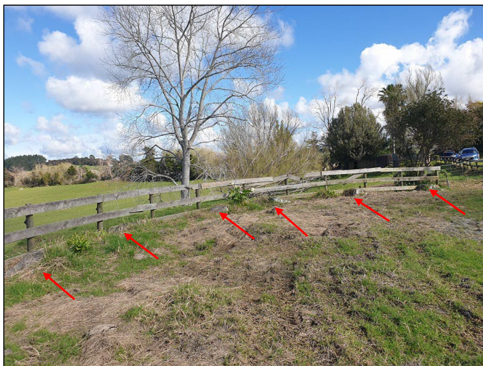
Figure 46. Concrete blocks of unknown provenance
