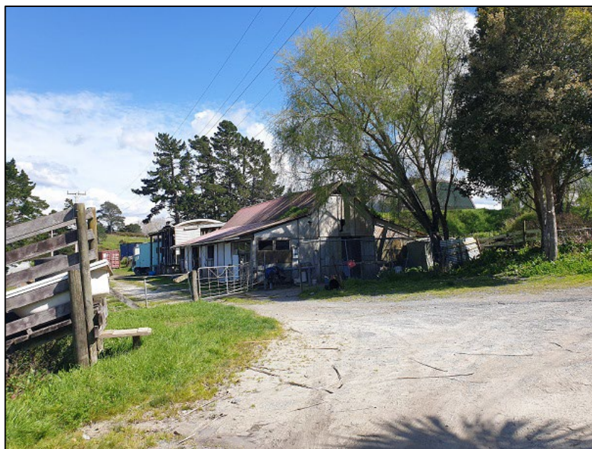
Figure 54. Stables and sheds located to the southwest of the house
