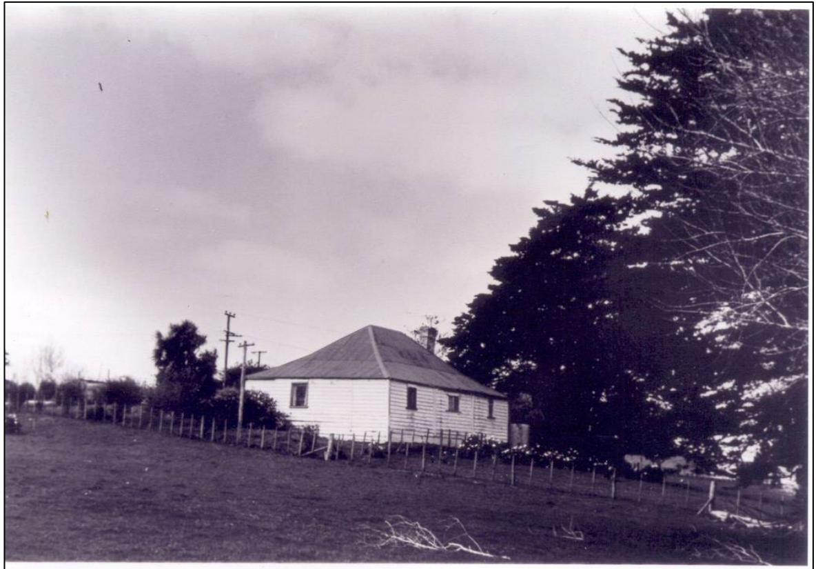
Figure 20 Photograph taken by Cecil Wright, and dated 1972, showing the rear (eastern and southern faces) of the house which is thought to have contained remnants of Maurice Kelly’s original homestead complex (source: 24.6.95, Silverdale & Districts Historical Society). Photo courtesy of Wainui Historical Society
