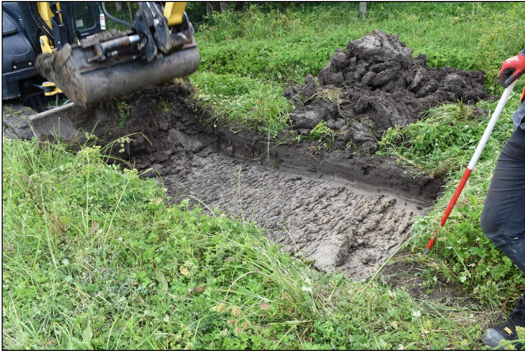
Figure 23 Photo of Trench 8 just before it was abandoned showing gleyed clay (facing northwest)
