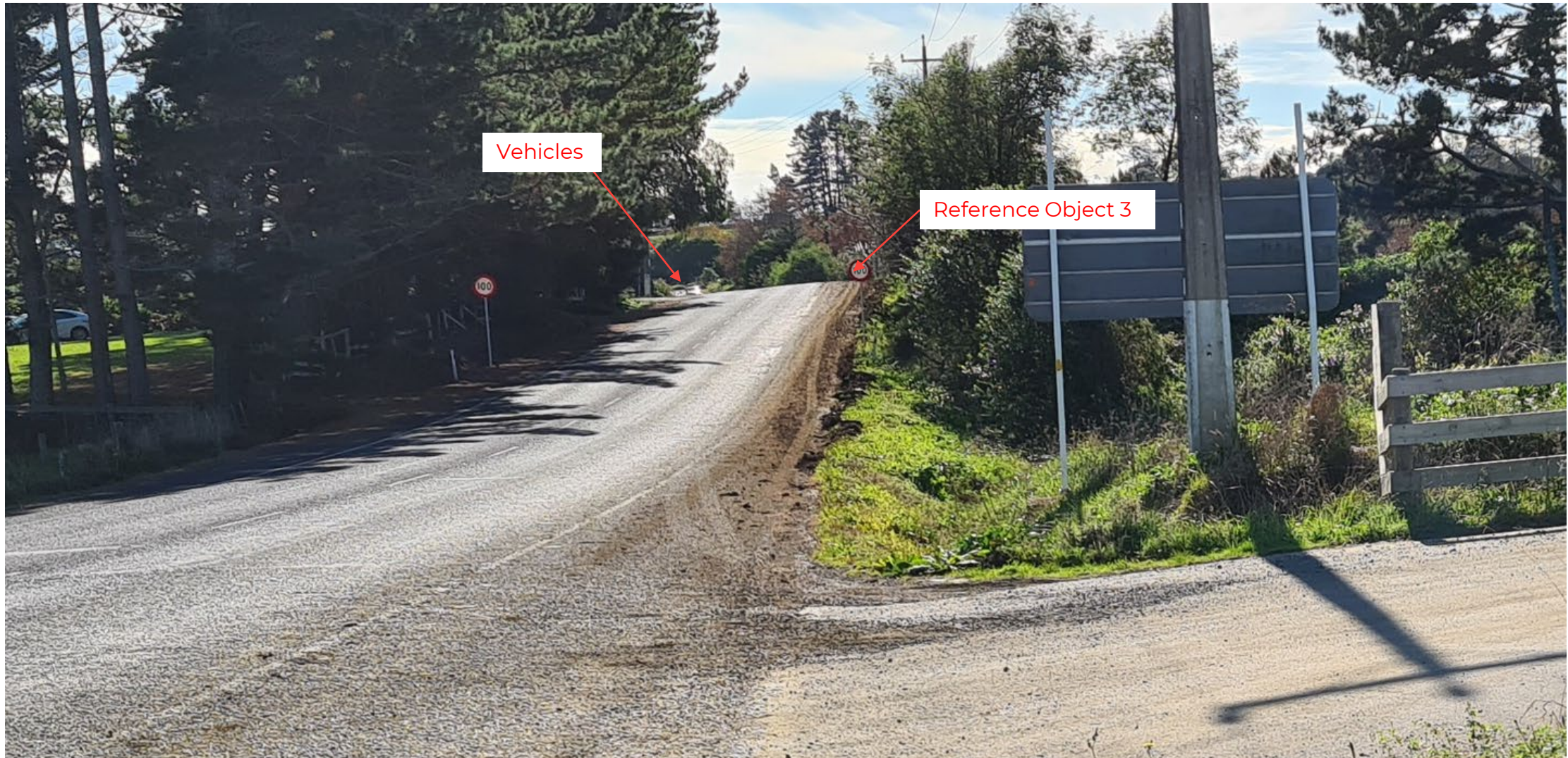
Visibility from the Site to Object 1 (To the north) The available sight distance between Object 1 and the proposed entrance is more than 233 meters
