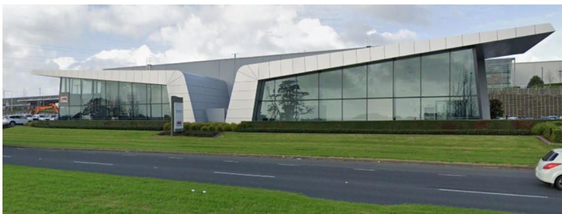
Figure 14: Example of the nature of architectural design outcomes anticipated through the application of design guidelines on sub-precinct A
