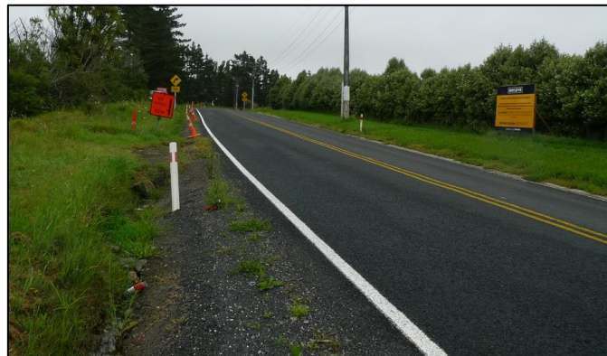
Figure 10: Trig Road looking South from the Proposed WBPPC's Roundabout Intersection
