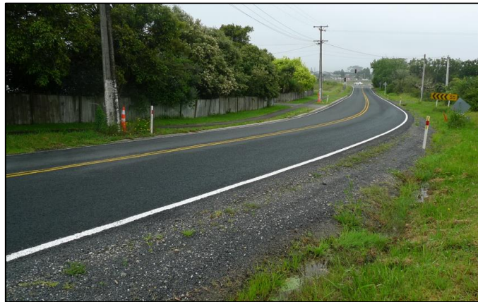
Figure 9: Trig Road Looking North from the Proposed WBPPC's Roundabout Intersection
