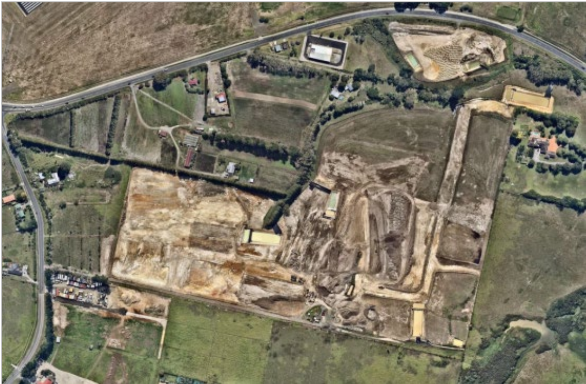
Figure 4: Bulk Earthworks Undertaken on Subject Site
