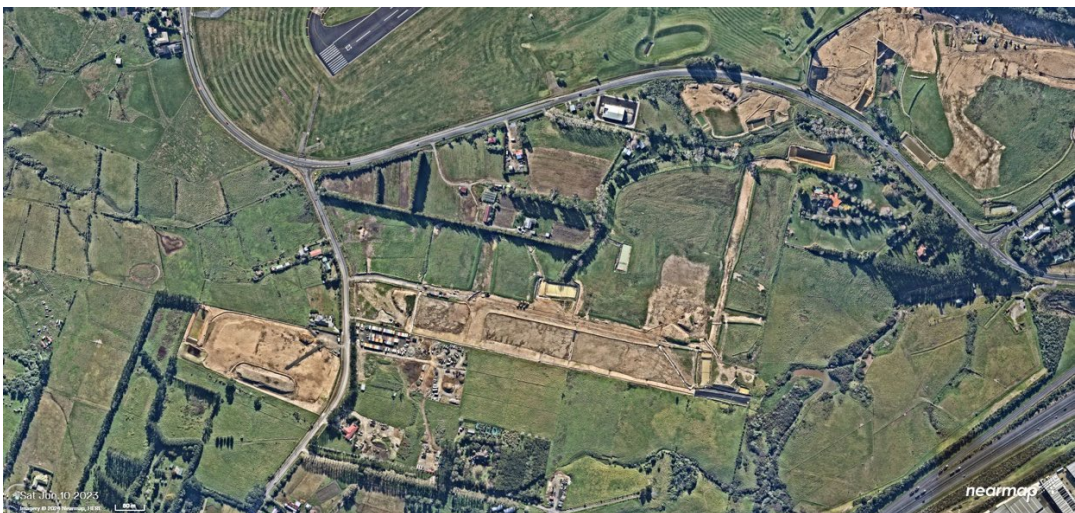
Figure 11: Aerial of earthworks 10 h June, 2023.
