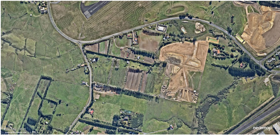
Figure 9: Aerial of earthworks 2 nd May, 2021
