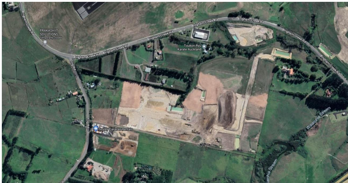
Figure 9 - Earthworks within the PPC land
