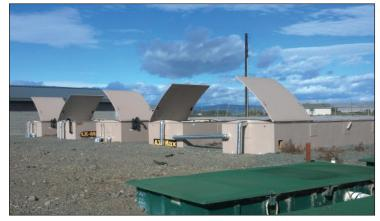
The Yakama Nations Housing Authority in Washington state added five AdvanTex<sup>®</sup> AX-Max units (background) to its ten AdvanTex AX-100 units, increasing the capacity of its wastewater system by 50%. Photo courtesy of Fextex Systems, Inc.
