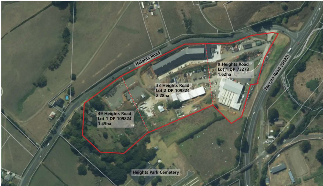
Figure 12: Existing hardstand areas (source: Google maps)
