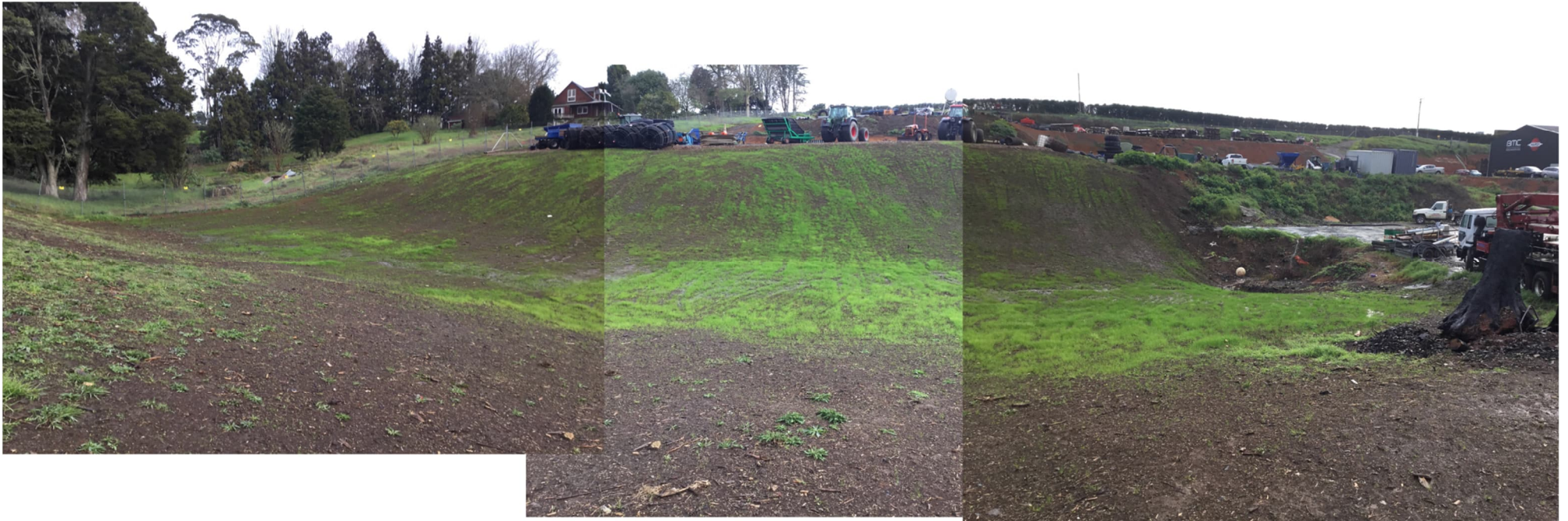
Plate 8. 33 Heights Road panoramic view taken from the southern side and showing part of 49 Heights Road (to the left) around to the lower part of 33 Heights Road (to the right). All trees and pasture shown within the red dotted polygon on Figure 1 have been removed and the area converted to hard-stand and landscape shallow gully (within which the overland flow path traverses).
