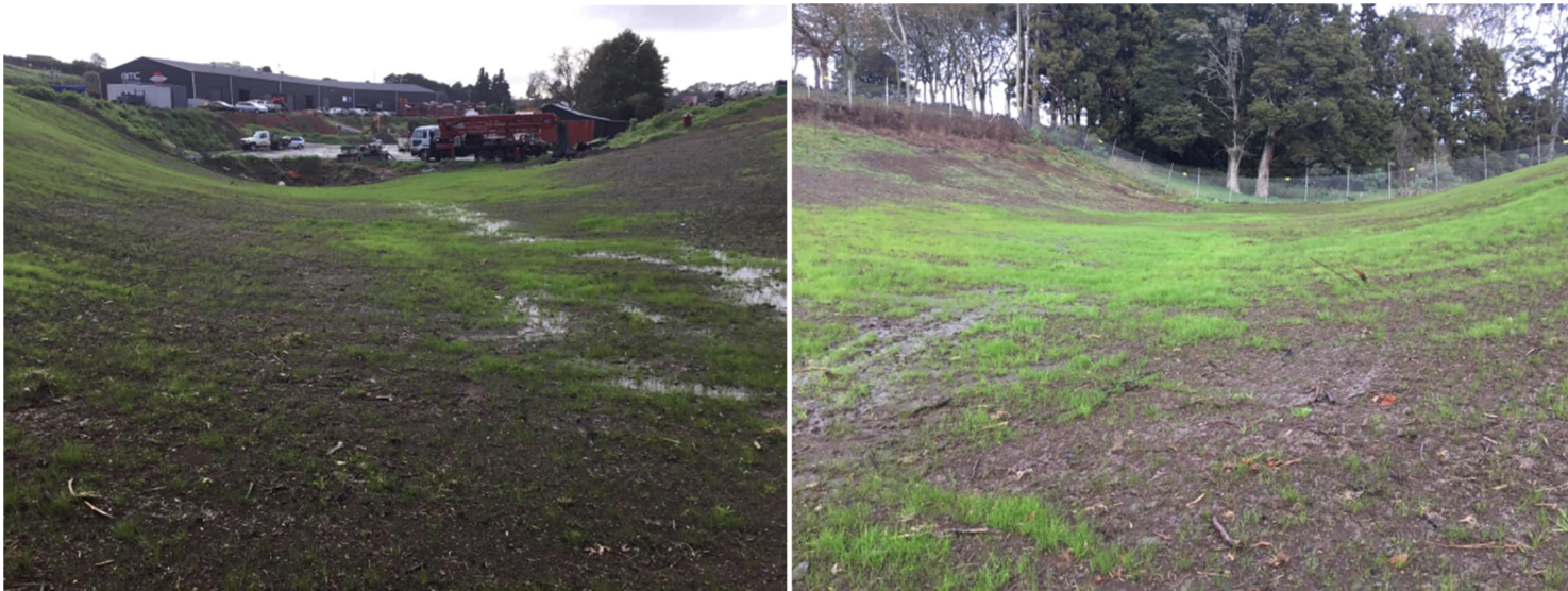
Plates 6 and 7. 33 Heights Road western end showing recent landscape works in the shallow gully (left photo looking down gully into 33 Heights Road after heavy rain; right photo looking up the shallow gully towards 49 Heights Road after heavy rain). Grasses establishing within landscaped areas are ryegrass and kikuyu.
