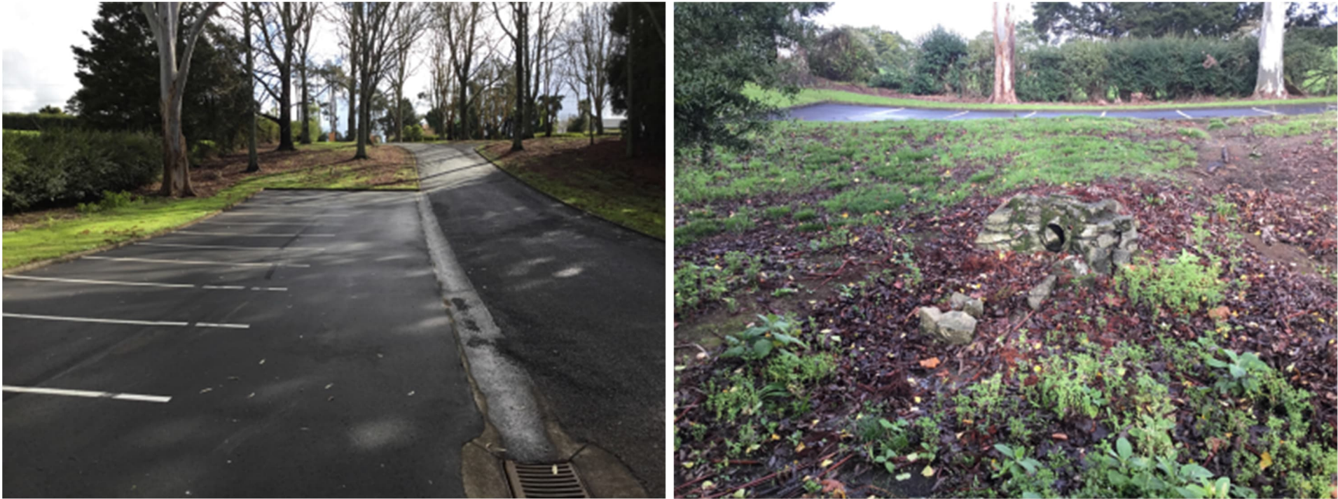
Plates 12 and 13. Cemetery adjoining 49 Heights Road to the south with car parking and road areas (top left and right) contributing overland flow to the overland flow path through 49 Heights Road (bottom left – looking down-gully, and bottom right – looking up-gully). The overland flow path is piped further down under 9 and 33 Heights Road.
