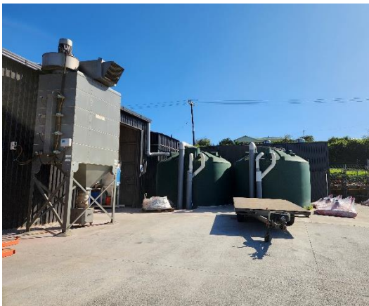
Figure 7: Stormwater tanks for the BMC Building
