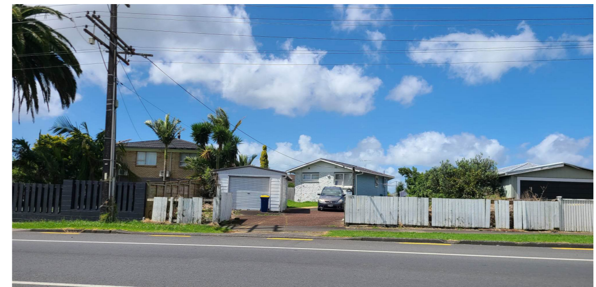
FIG 12 ADJACENT RESIDENTIAL BUILDINGS OPPOSITE HOBSONVILLE ROAD
