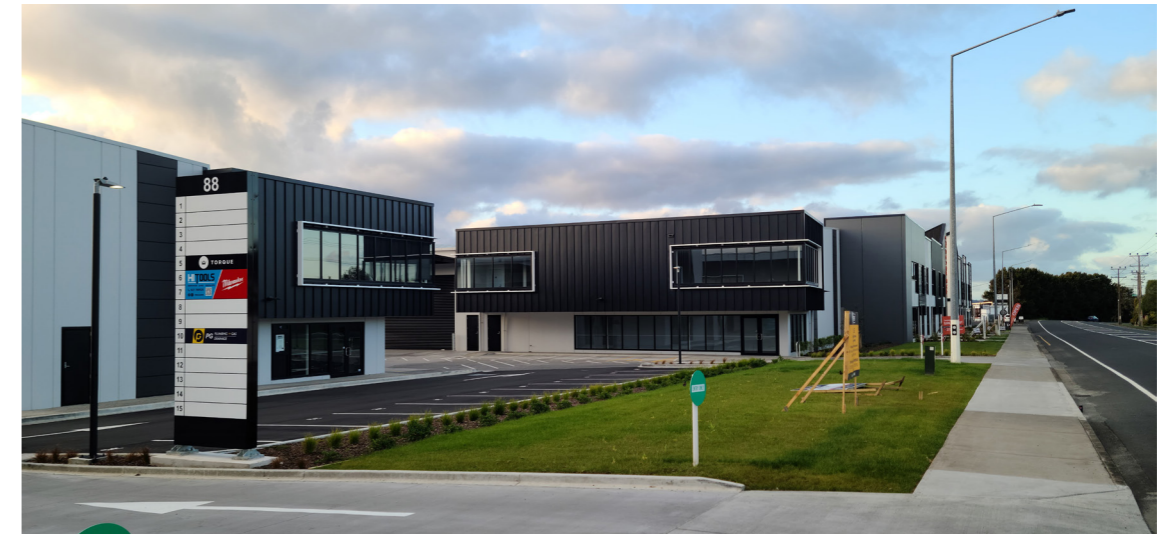
FIG 10 ADJACENT LIGHT INDUSTRIAL BUILDINGS
