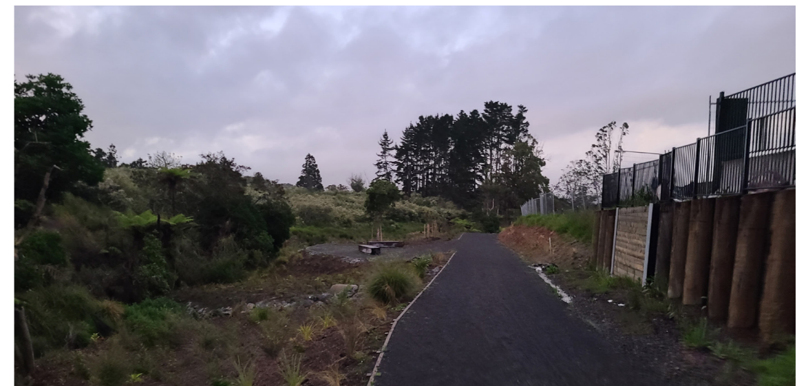
FIG 16 RAWIRI STREAM SHARED PATH, LOOKING NORTH. WESTPOINT DRIVE SITS TO THE RIGHT OF THE IMAGE.
