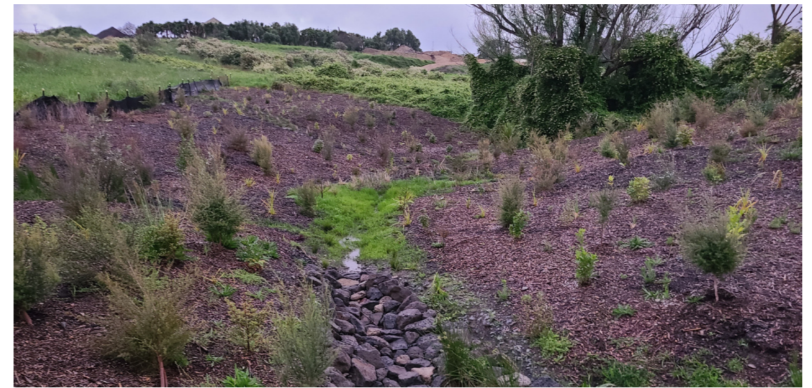
FIG 15 RAWIRI STREAM LOOKING TOWARD PRECINCT 1
