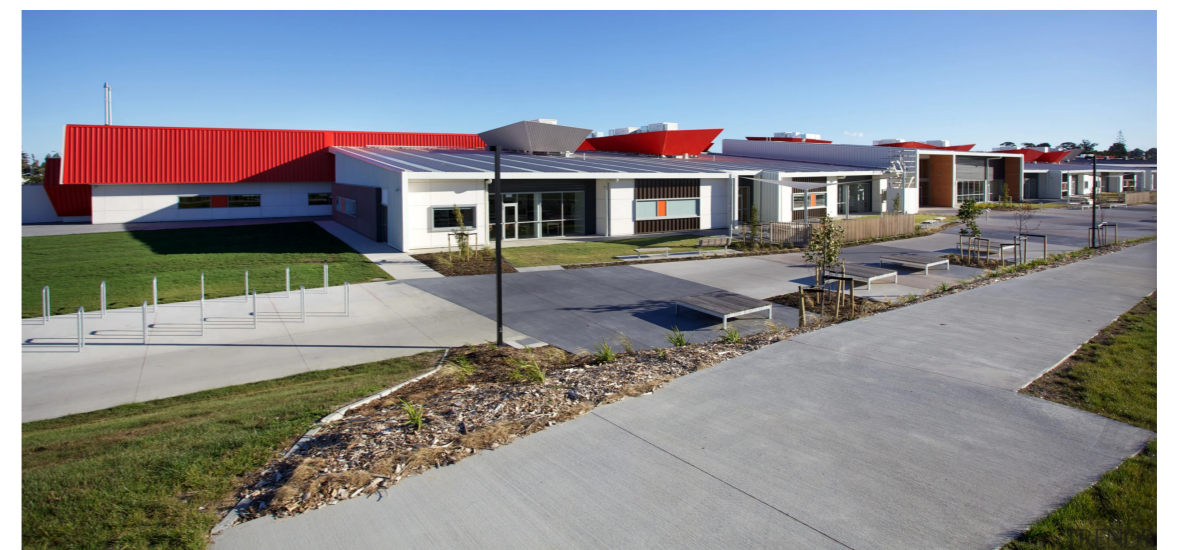
FIG 7 HOBSONVILLE SECONDARY SCHOOL (SOURCE: MINISTRY OF EDUCATION WEBSITE)
