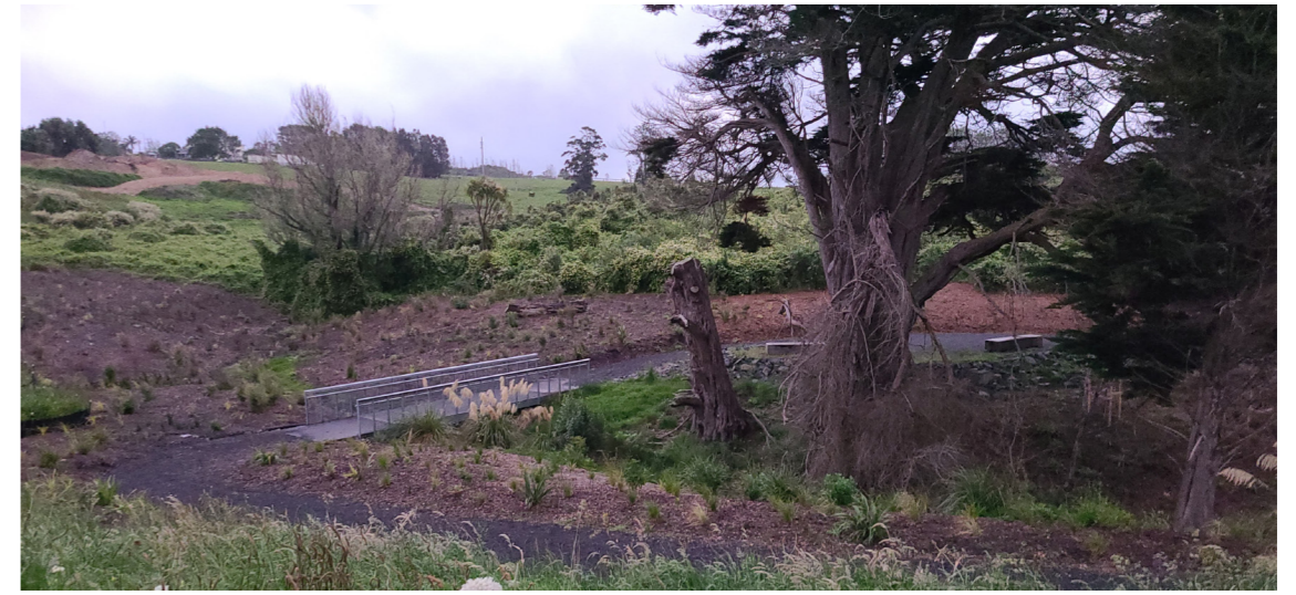
FIG 14 RAWIRI STREAM FOOTBRIDGE, LOCATED ADJACENT TO BLOCK 1
