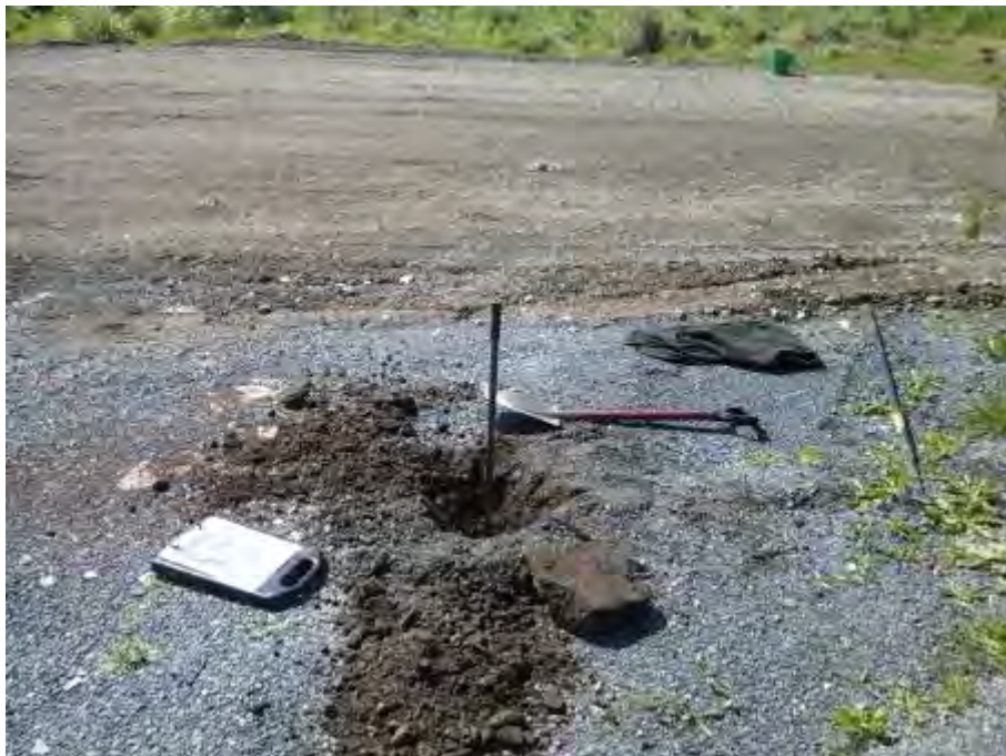
PLATE 4: Overlooking SS6, located under compacted gravel
