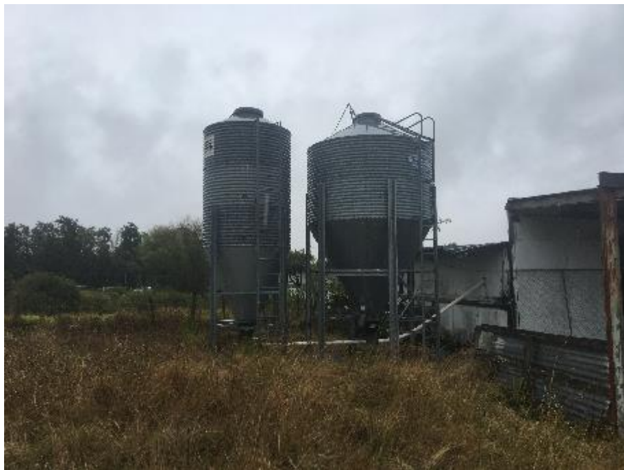
PLATE 4: GRAIN SILOS ON SOUTHEAST CORNER OF POULTRY SHED
