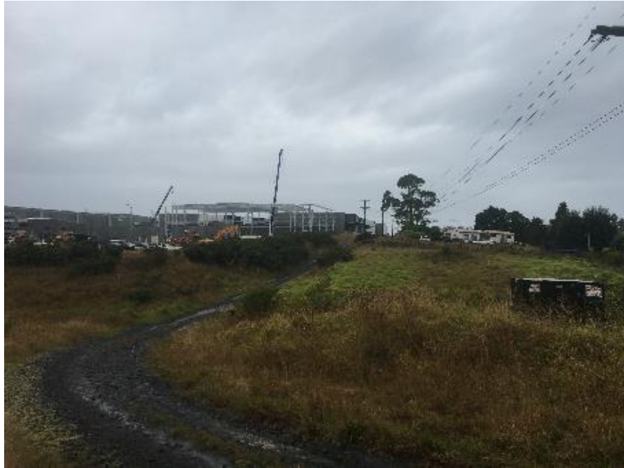
PLATE 1: ACCESS ROAD ALONG NORTHERN BOUNDARY OF 100 HOBSONVILLE ROAD
