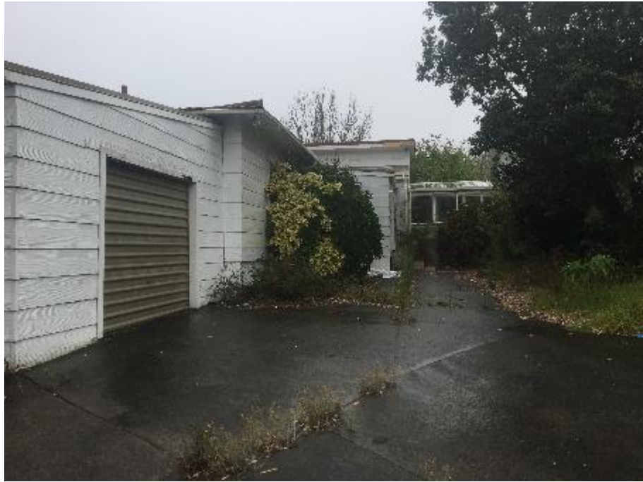
PLATE 7: ORIGINAL DWELLING WITH MODERN GARAGE EXTENSION IN FOREGROUND
