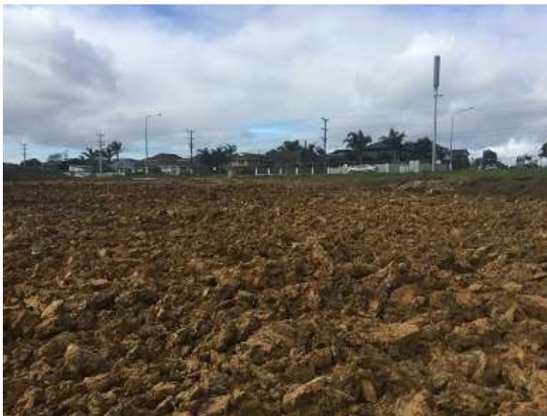
Photo of site showing south-eastern fill area.
