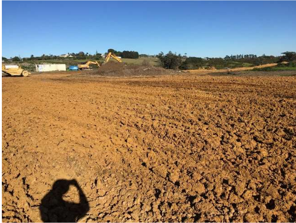
Fill progress in north-eastern corner.
