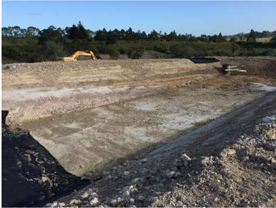
Photo of site showing new sediment pond in north-western corner.
