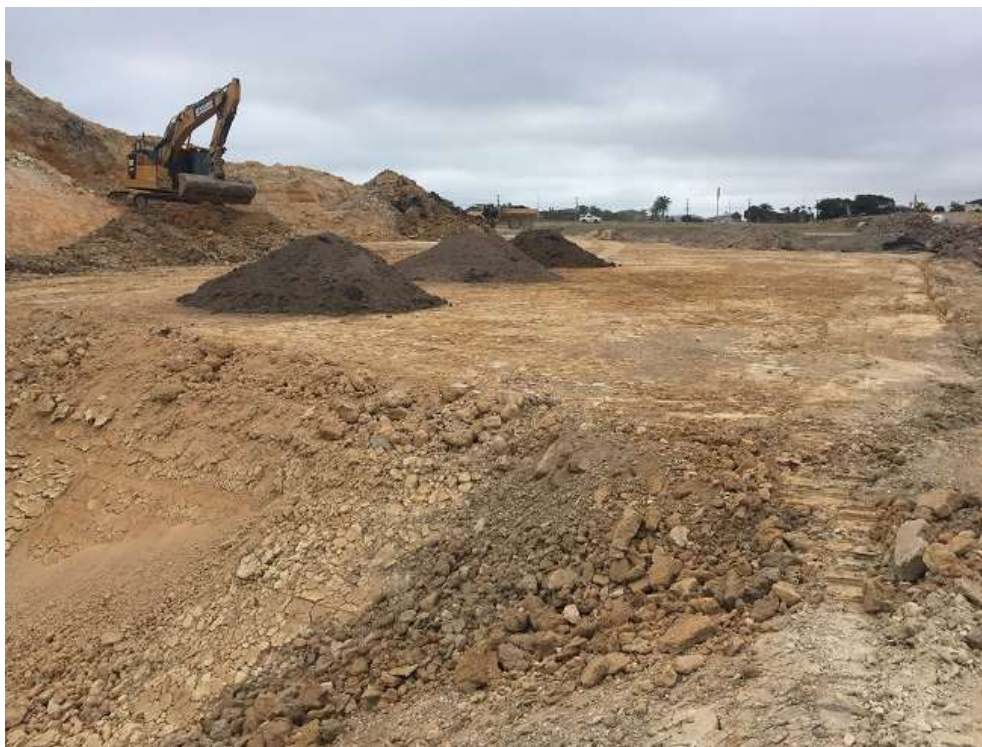
Trimmed fill surface on 27/01/21.
