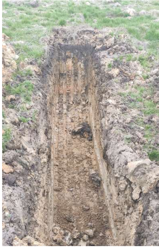
Figure 7 - Western end of test pit 2 (competent fill).
