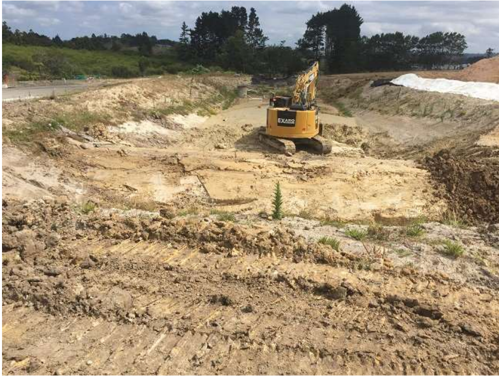
Part of southern part of pond stripped.
