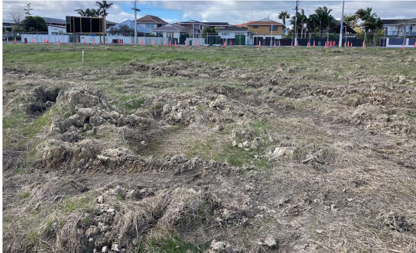
Figure 3. Photo taken looking towards Lot 4 with similar rutting evident.
