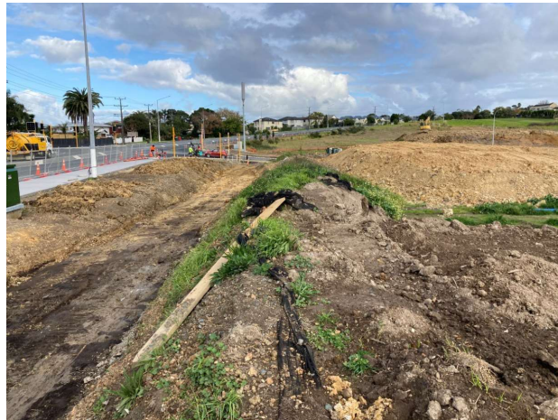
Photo of haul road on Lot 5 looking to the south
