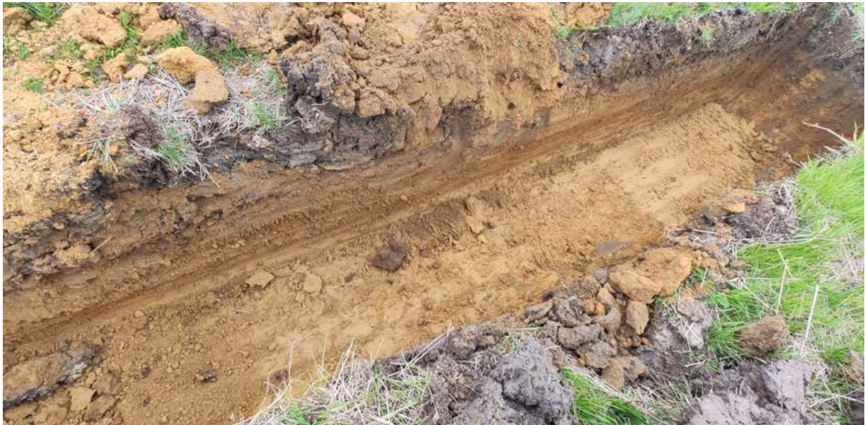
Figure 5 - Test Pit 5 (No Weak Fill)
