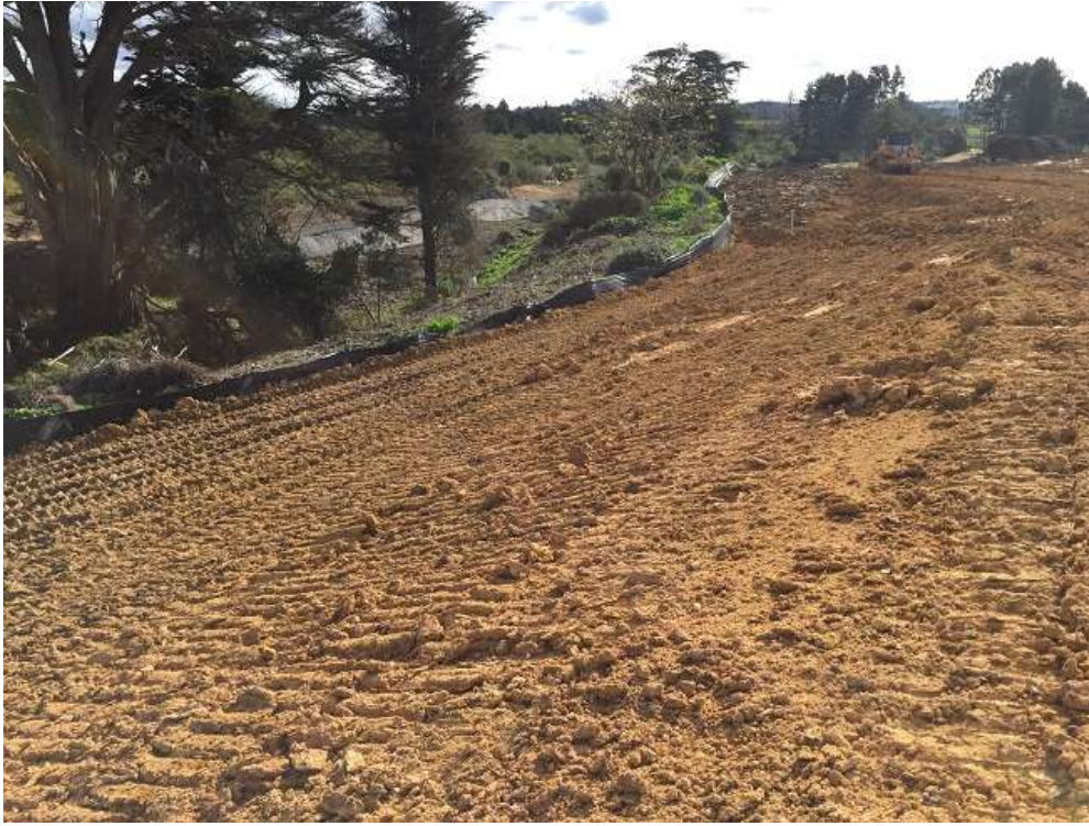
Extent of fill placed near western boundary.
