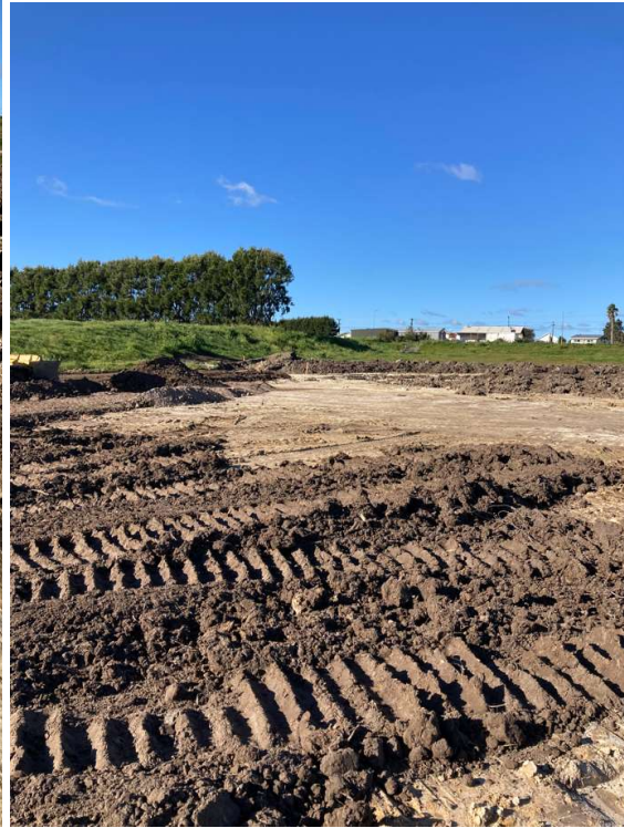
Stockpile fully removed from Lot 10.
