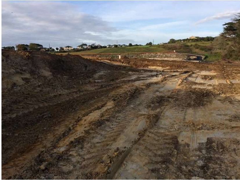
Photo of site showing cut area after additional stripping since yesterday.
