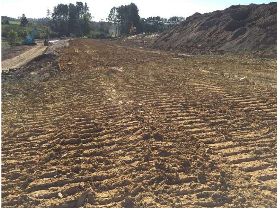
Filling along western boundary under approx. future Spine Rd carriageway.
