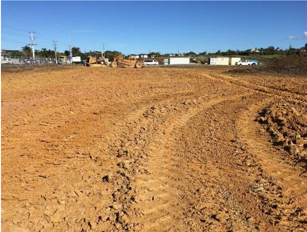
Fill progress in north-eastern corner.
