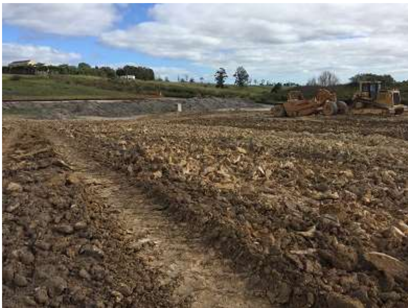
Photo of site showing site conditions at time of inspection.
