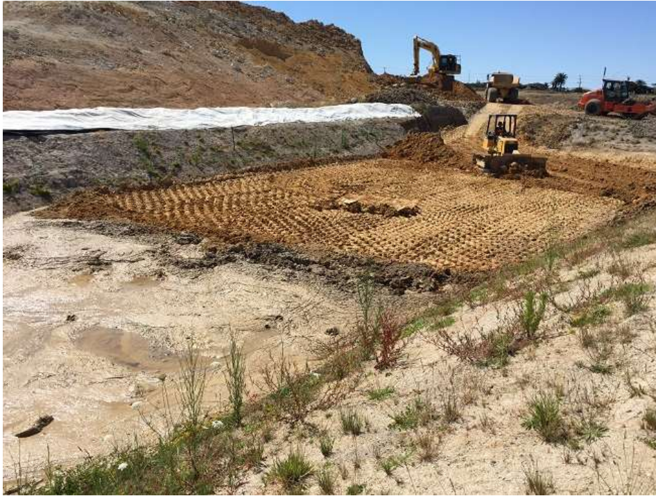
First lift of fill in the southern end of the pond.
