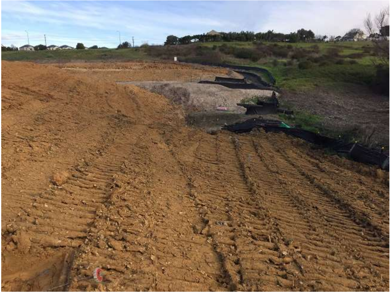
Fill progress near the western boundary, north of the southern pond.
