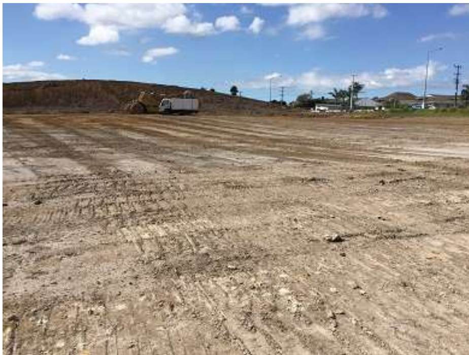
Photo of site showing the dry south-eastern stripped area.
