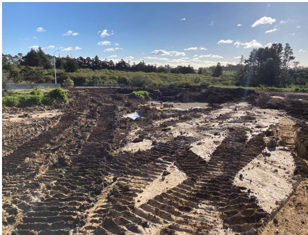
Looking at the decant pond in the north-western corner of Lot 10.
