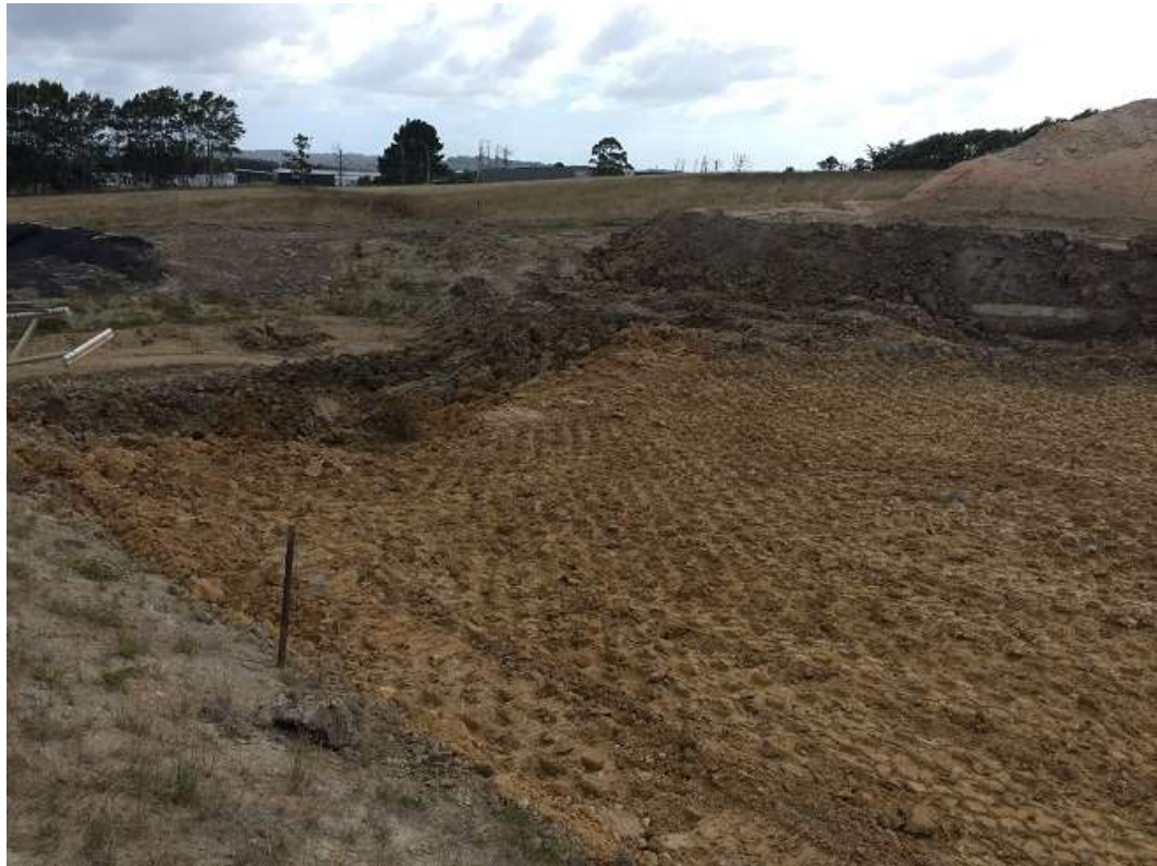
Fill placed in the southern end of the pond.
