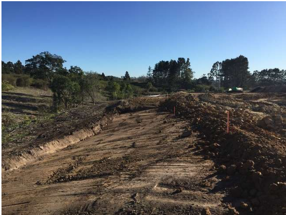
Stripping along western boundary under approx. edge of Spine Rd carriageway.
