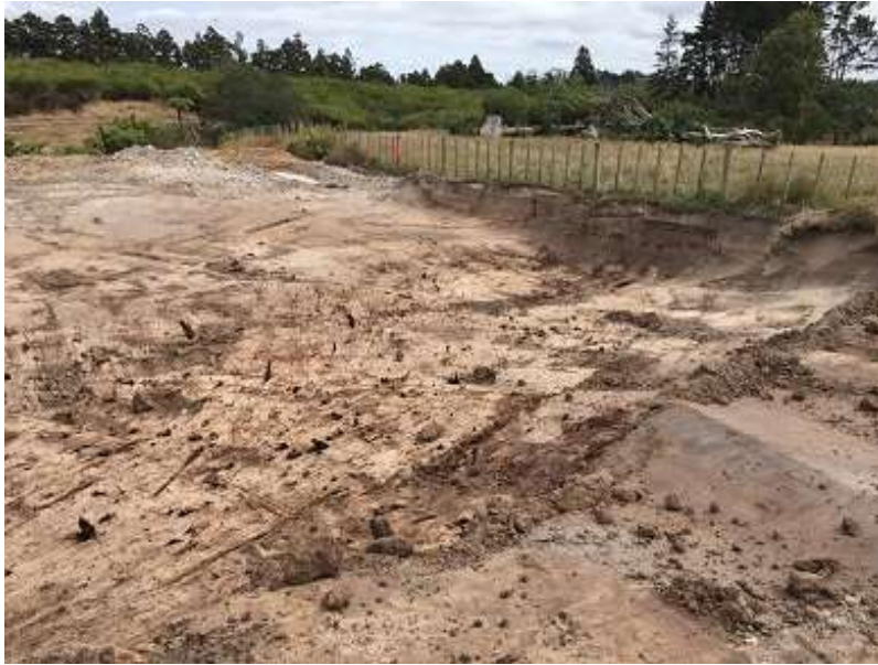
Photo of site showing stripped north-western area.
