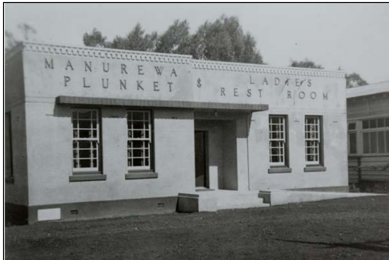
Figure 7. 11 September 1945 – newly built Manurewa Ladies Plunket and Restroom. Manukau Research Library, MCP: I, 5, no.7. Footprints 01600. Courtesy of Wichman, G.
