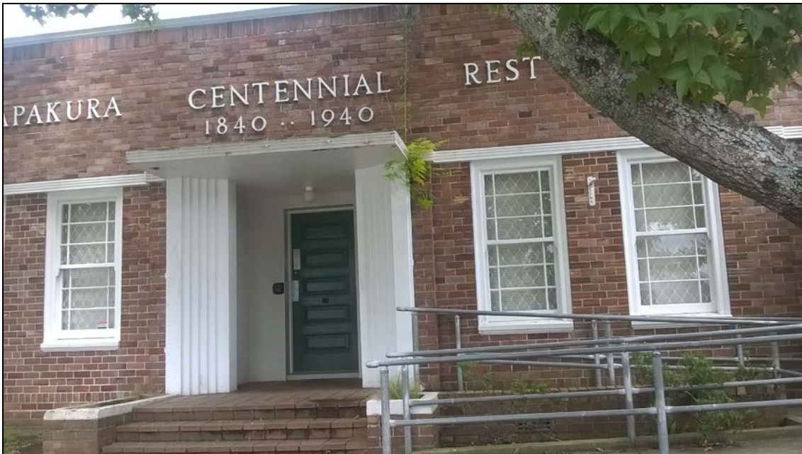
Figure 42. Zoomed-in view of front elevation of the building, with later metal ramp.
