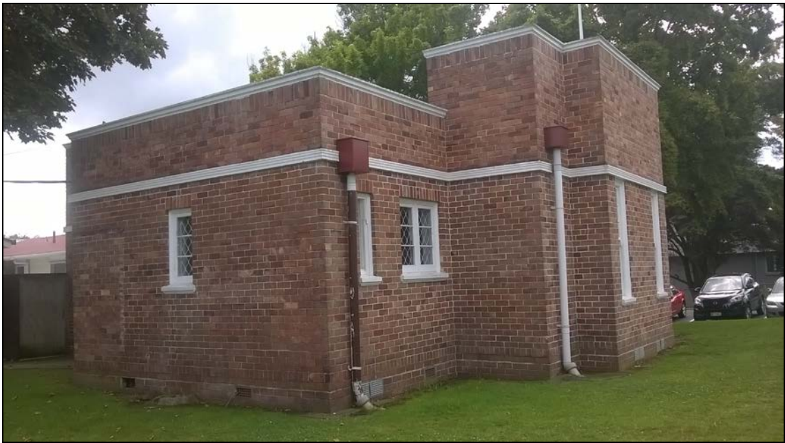
Figure 45. Side and rear elevation of the restroom.
