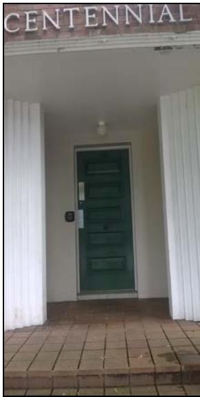
Figure 54. Front portico entrance
