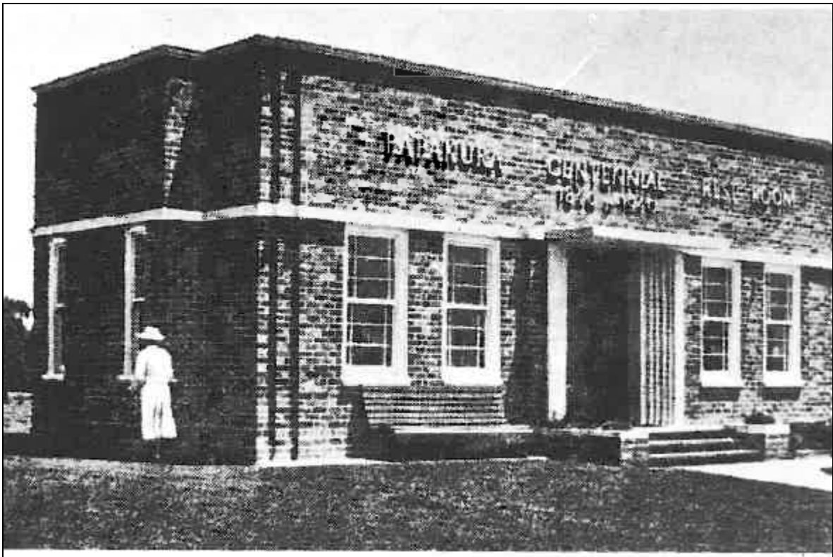
Figure 20. Front and side image of the restroom building. A park bench was present in front of the building at that time (date of image unknown). Yousef, R. (1997). p 18.
