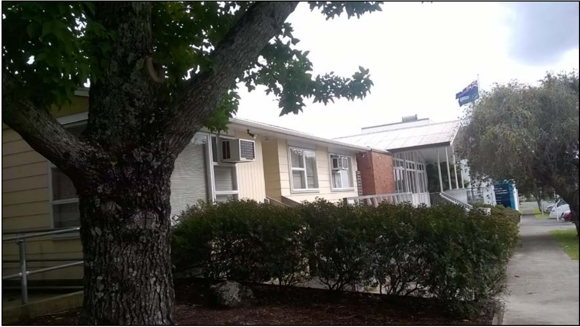
Figure 49. Next door council buildings.
