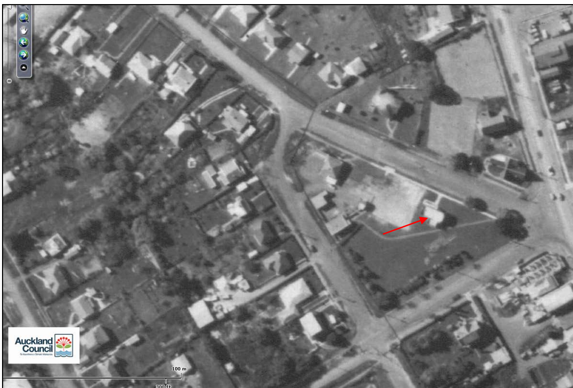
Figure 4. c. 1959 aerial of site and immediate surrounds. AC, GIS 2010-2011.
