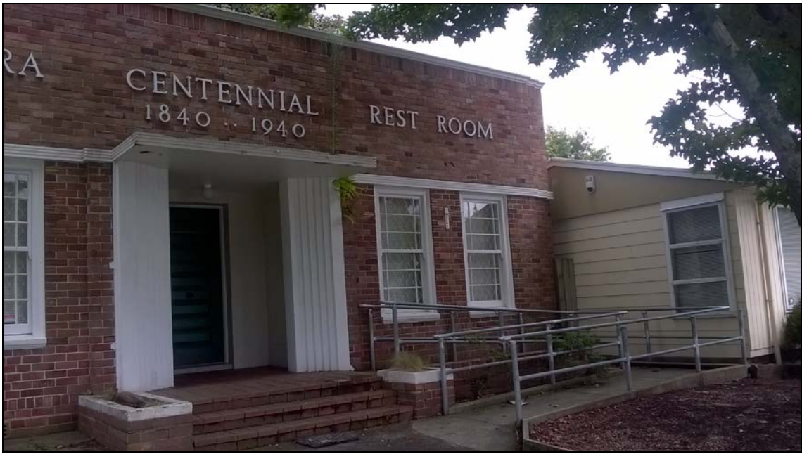
Figure 43. Front elevation with the pre-fabricated Council building hard up against the side of the subject building.
