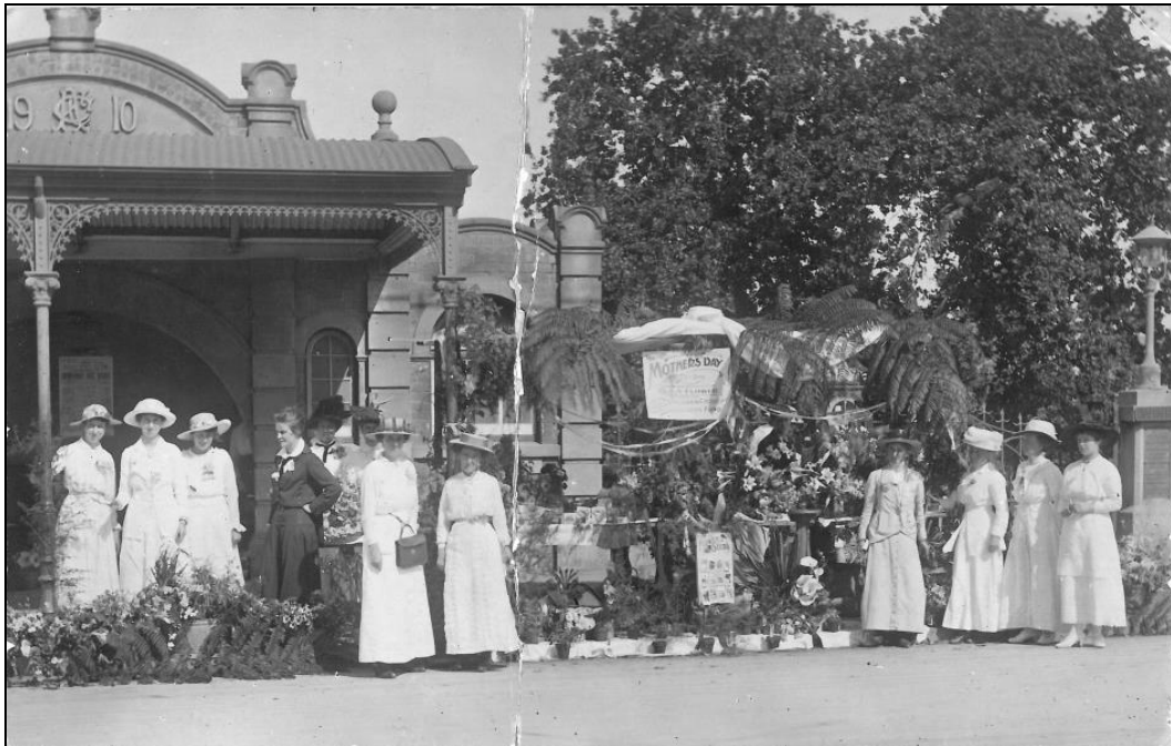
Figure 10. Photograph of the Mother's Day celebrations in front of the newly constructed womens toilets'. c. May 1910. Reference: Sir George Grey Collection 1037-1.
