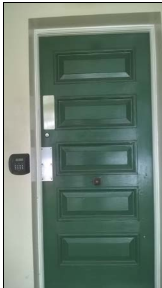
Figure 55. Five panel timber front door remains (likely original)
