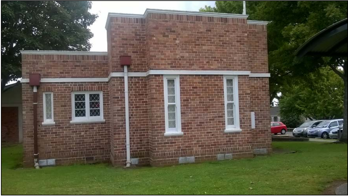
Figure 47. Side elevation of the building, as seen within the park.
