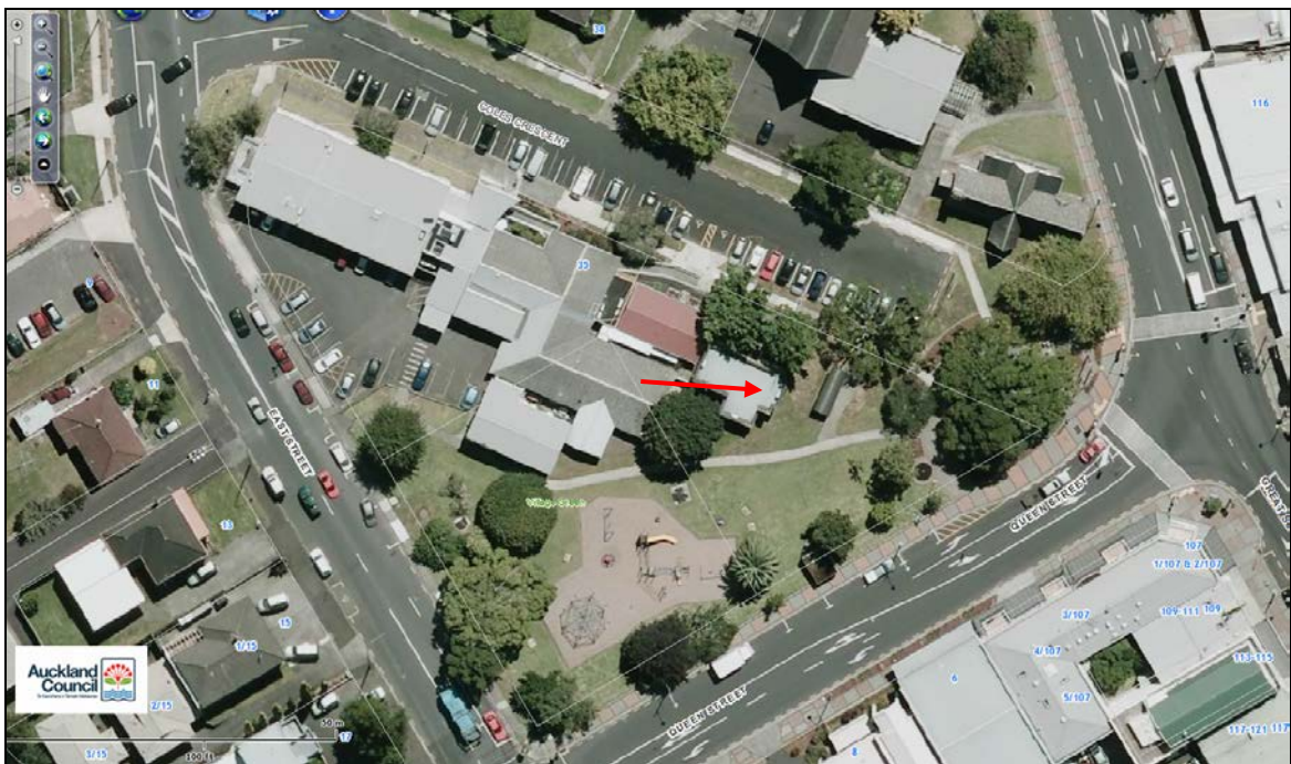
Figure 2. Aerial of restrooms and Plunket building in the context of 35 Coles Crescent site. AC, GIS 2010-2011.
