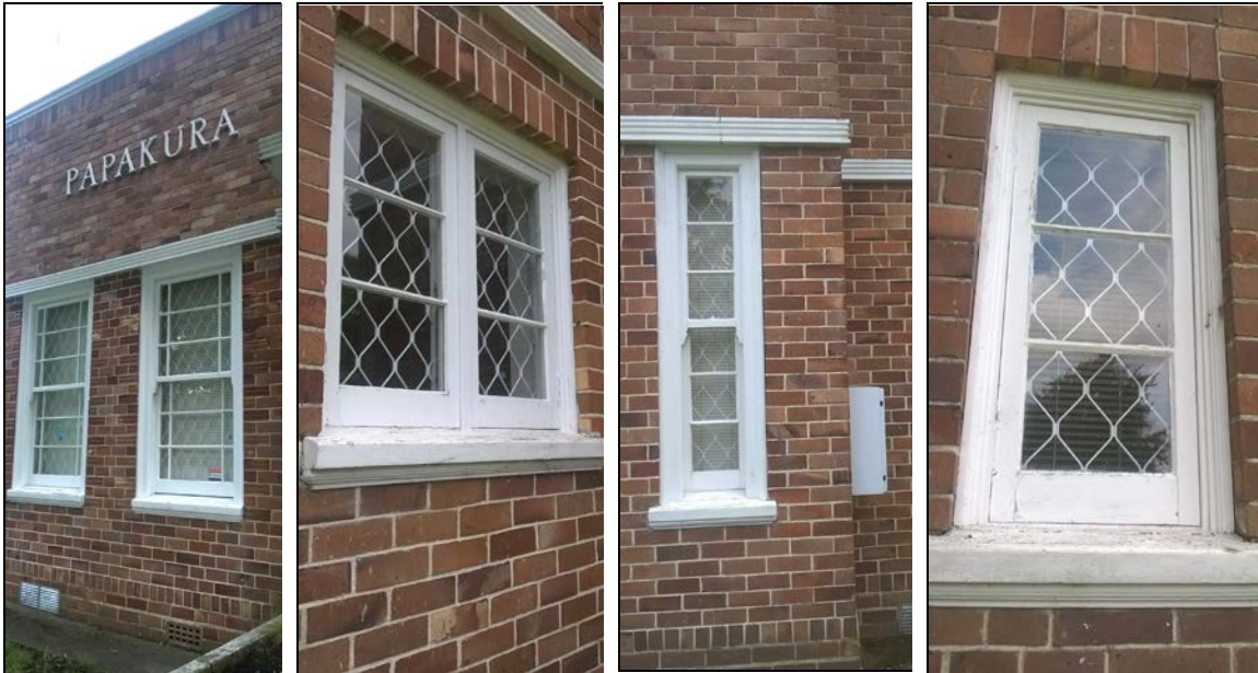
Figures 50-53. Exterior of windows. Front elevation windows are the original double-hung timber framed windows.
