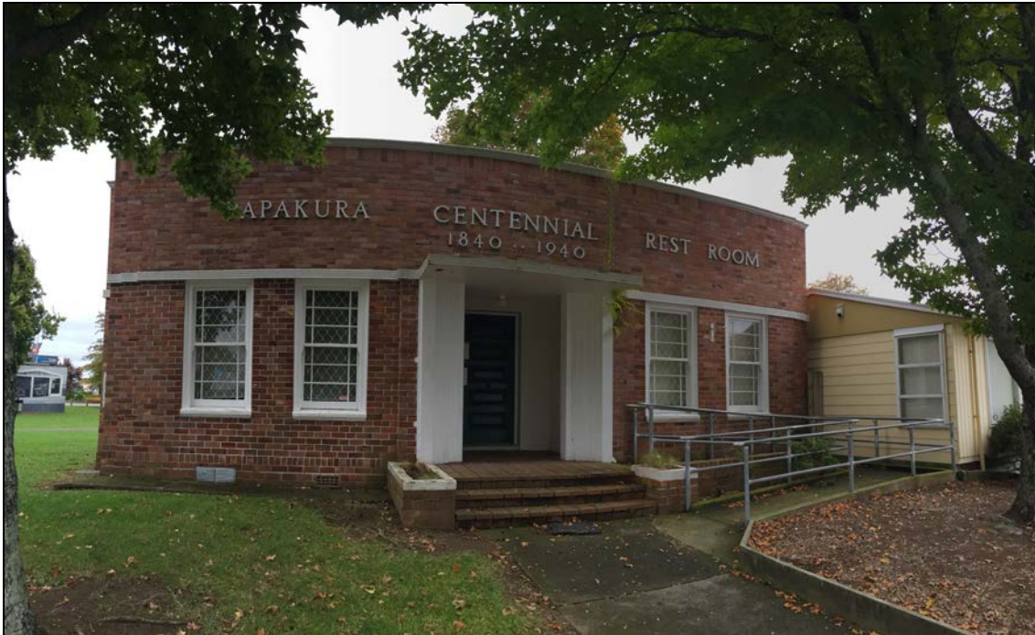
Figure 41. Front elevation of building, with prefabricated building nearby in right side of frame.
