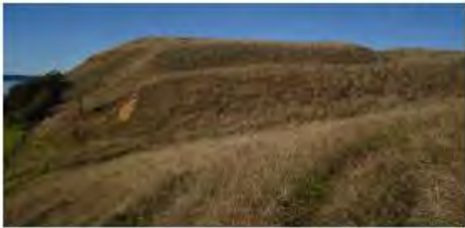
Plate 8. Western external terrace
