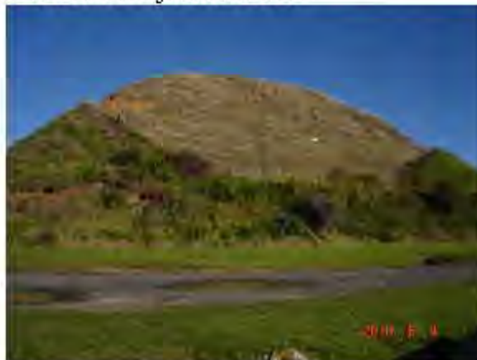
Plate 2. Looking from the northeast. Erosion and some slumping visible.
