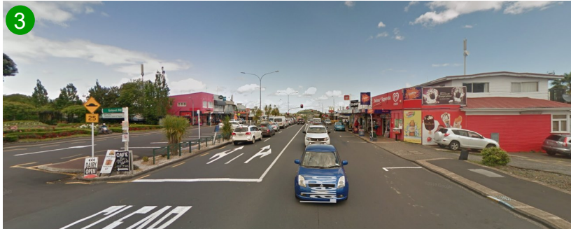
ABOVE FIG. 2-20: Lake Road at the School Road junction: two southbound lanes, one northbound lane, parking and a footpath on the west side, a southbound slip road with parking, a bus stop, and a footpath on the east side.
