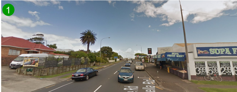
ABOVE FIG. 2-18: Lake Road at the Corrella Road intersection: one general vehicle lane in each direction, parking on the west side, a southbound cycle lane on the east side and footpaths on both sides.
