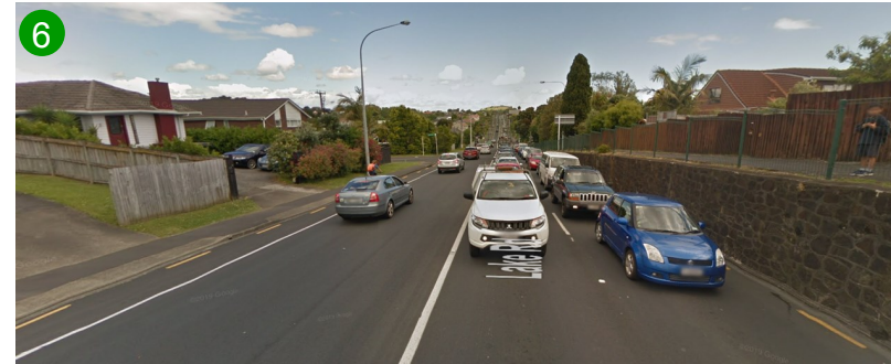
ABOVE FIG. 2-23: View of the Lake Road south of the centre: two southbound lanes merging, two northbound lanes, cycle lanes in both directions and footpaths on both sides; the road is relatively steeply sloping to the south.
