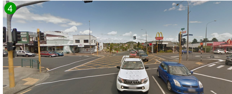
ABOVE FIG. 2-21: The Lake Road-Bayswater Avenue intersection: two southbound lanes, two northbound lanes merging, and a free left turning lane out of Bayswater Avenue (right); the slip road entering onto Williamson Avenue (right).
