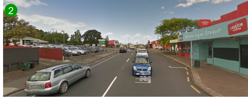
ABOVE FIG. 2-19: Lake Road at the Egremont Street intersection: one general vehicle lane in each direction, indented parking on the west side, a southbound cycle lane on the east side and footpaths on both sides.
