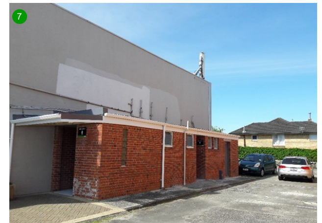
ABOVE FIG. 2-13: Public toilets between the barber shop and the liquor store east of the slip road.
