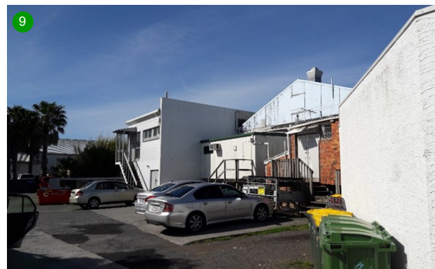
ABOVE FIG. 2-15: Service area behind the shops on the west side of Lake Road.
