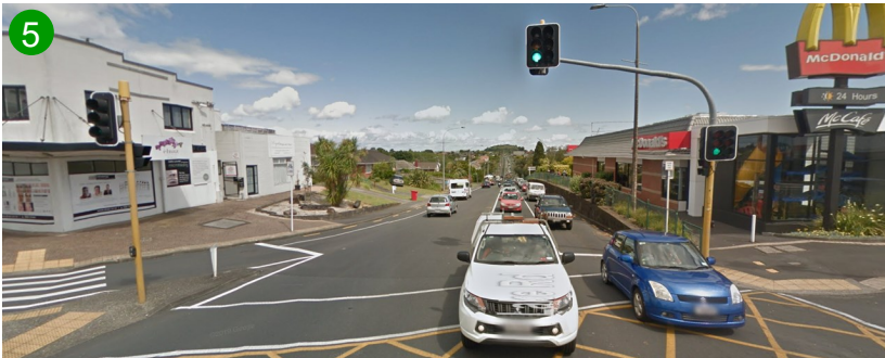
ABOVE FIG. 2-22: View of the Lake Road-Bayswater Avenue intersection: two southbound lanes merging, two northbound lanes, and a free left turning lane out of Williamson Avenue (left).
