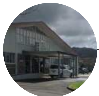
Community hall porch. Loading and unloading protected from the rain.
