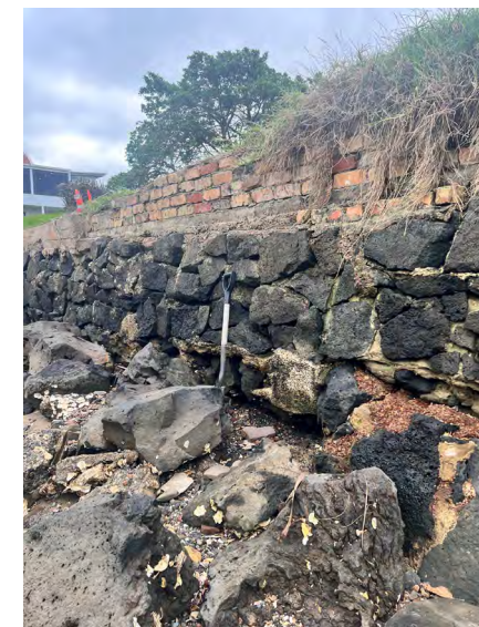
Stage 3: Undermined Rock masonry walls on the beachfront and into the stream mouth.
