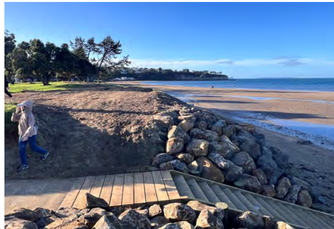
Renewed Revetment structure at Southern-end.
