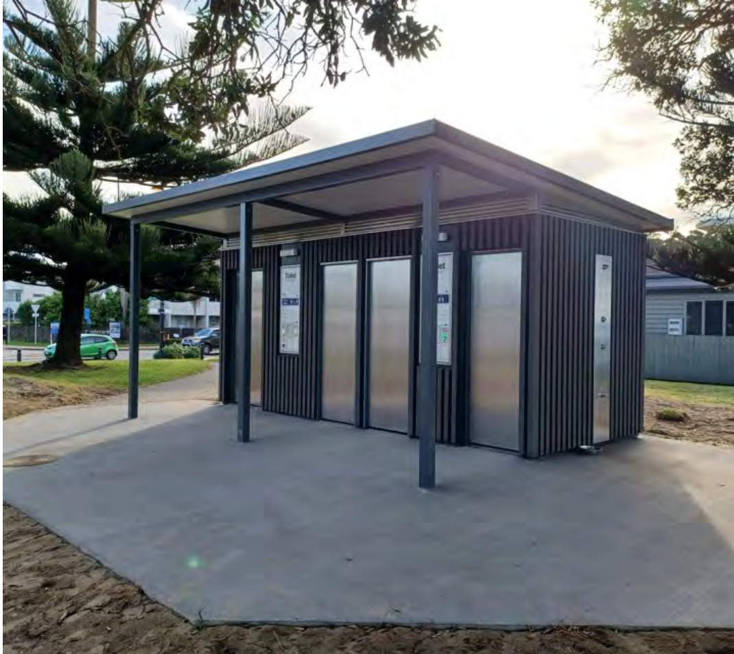
Toilet Renewal at Orewa Reserve – Facility open a of July 2024
