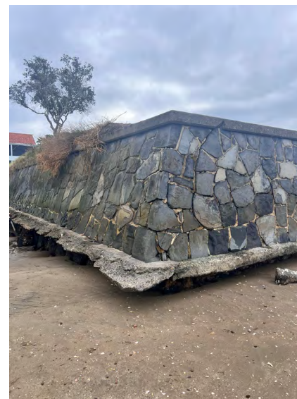
Stage 3: Undermined Rock masonry walls on the beachfront and into the stream mouth.
