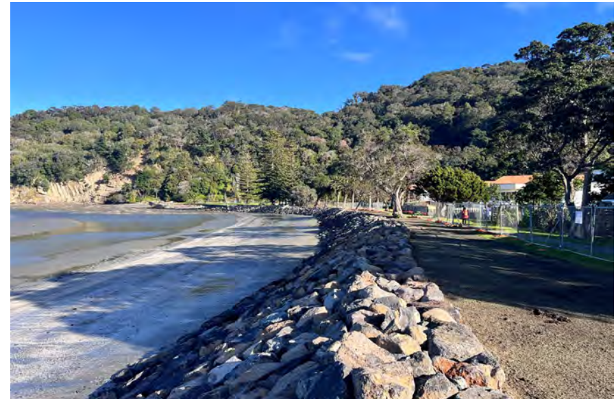
Renewed Seawall at completion. (July 2024)
