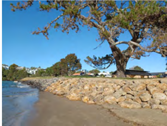
Renewed Revetment structure near toilet block
