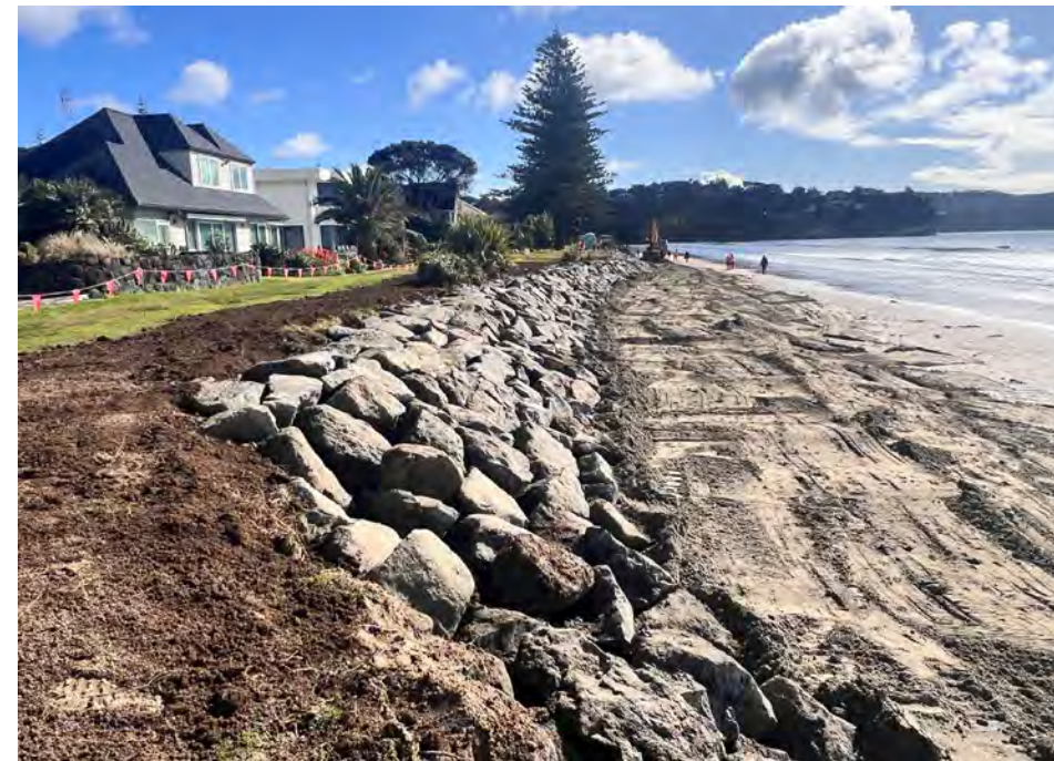
Renewed Seawall in Stage 2 at completion. (August 2024)
